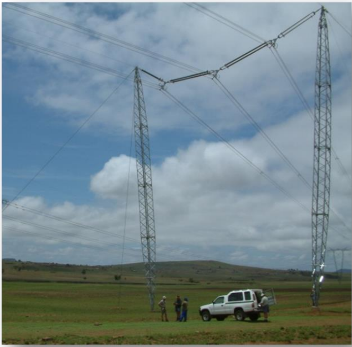
Plate 1: Cross Rope Tower
