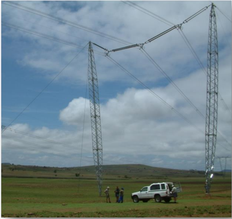
Plate 1: Cross Rope Tower
