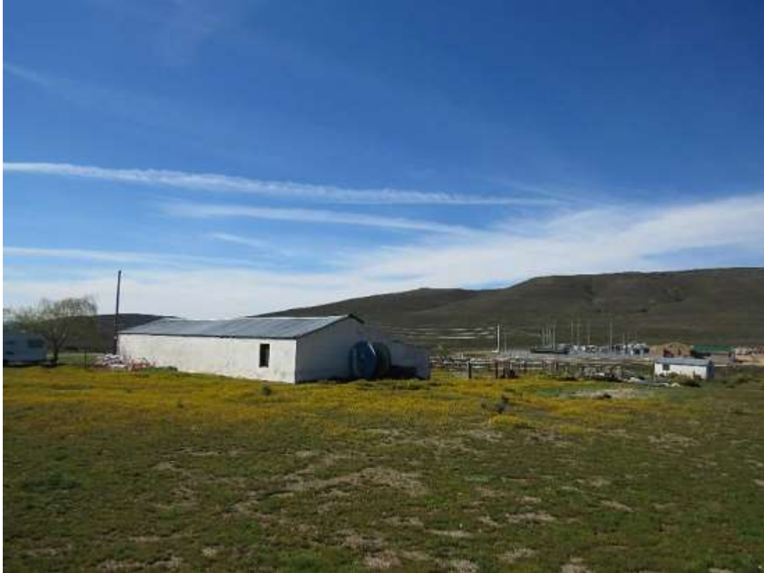
Figure 3-7: Bon Espirance substation under construction (source: SiVEST, 2021)
