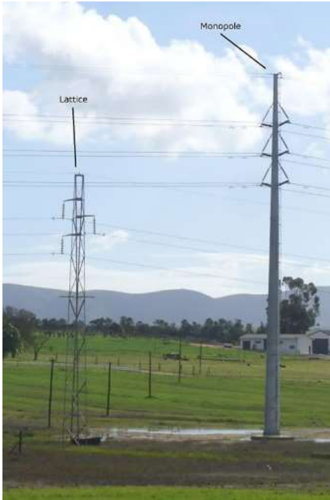
Figure 3-6: Conventional lattice powerline tower compared with a steel monopole structure
