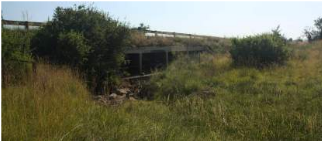
Figure 6: View of the seasonal stream 3 in the northern portion of the pipeline route. The stream will be crossed by the pipeline and is in a good condition, utmost care must be taken to keep the impact on the stream to a minimum.
