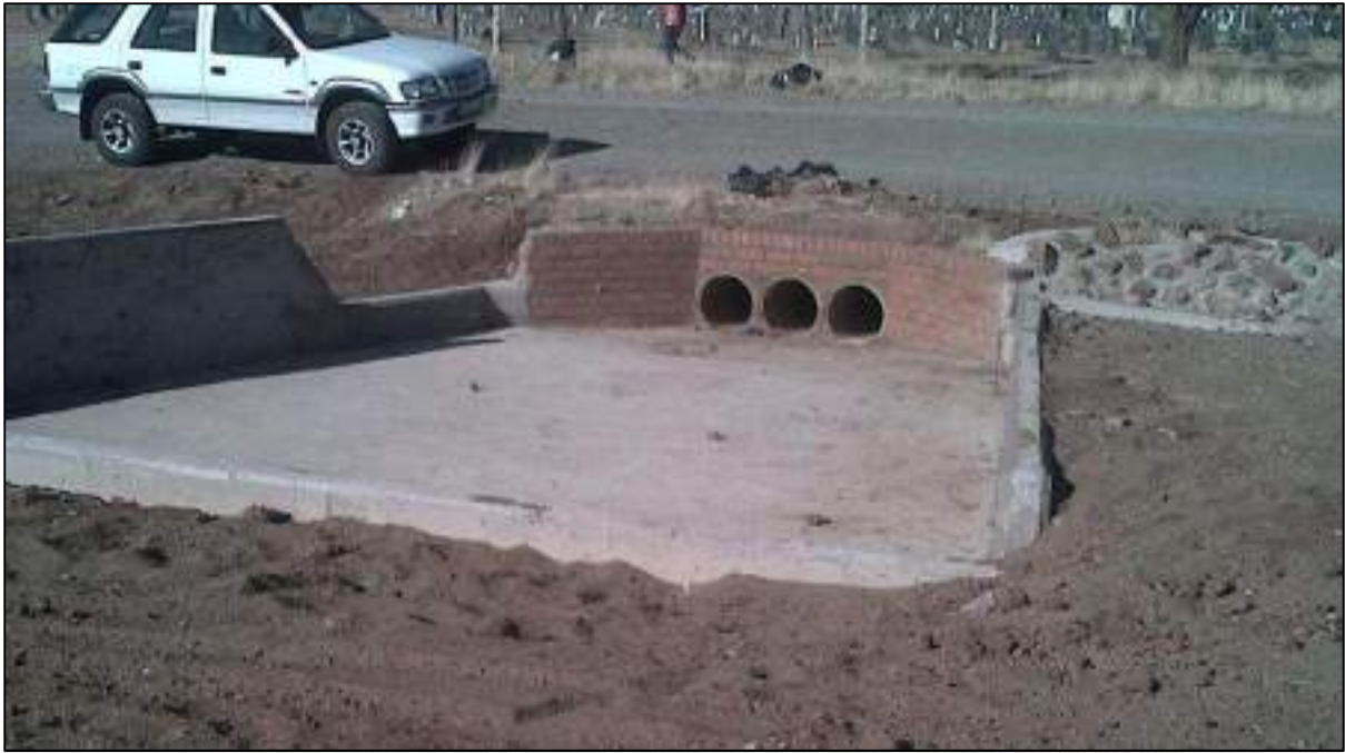
Example of a stream cross protection measured that will be implemented to protect the pipeline as well as to limit possible erosion.
