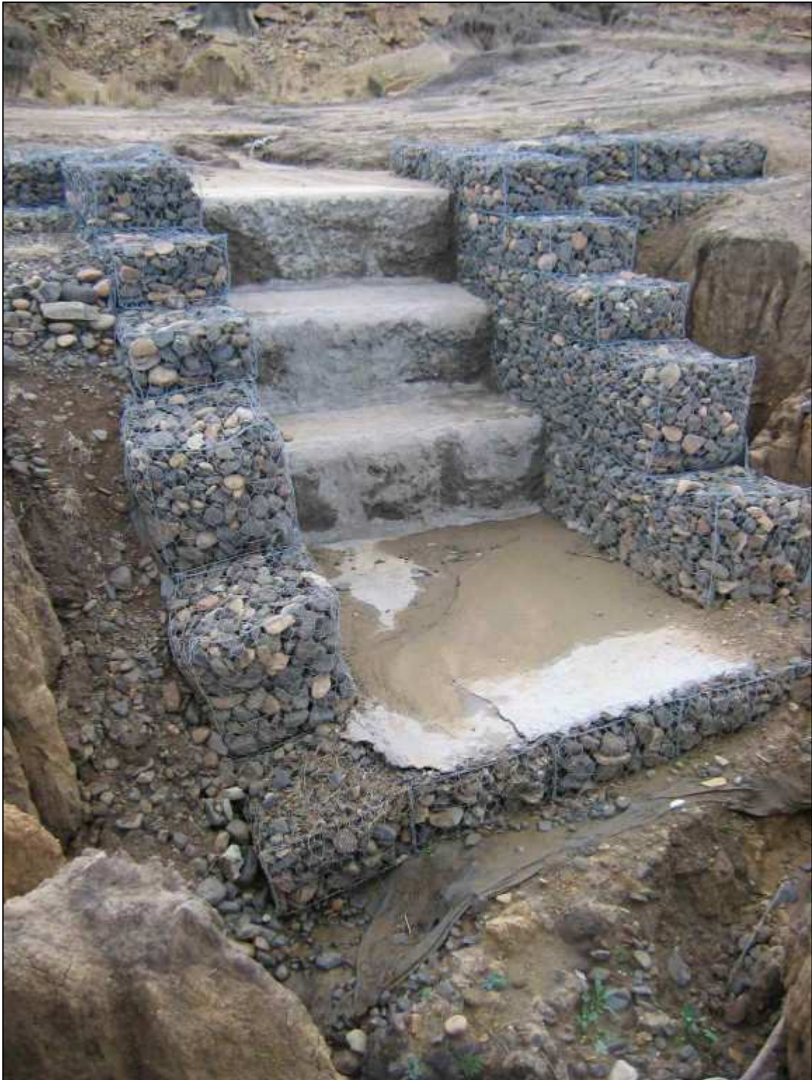
Example of a gabion constructed as part of a stream cross protection measures to be implemented
