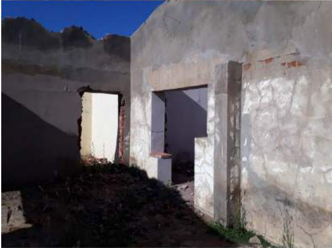
Figure 9. Modern alterations, interior of the main house.
