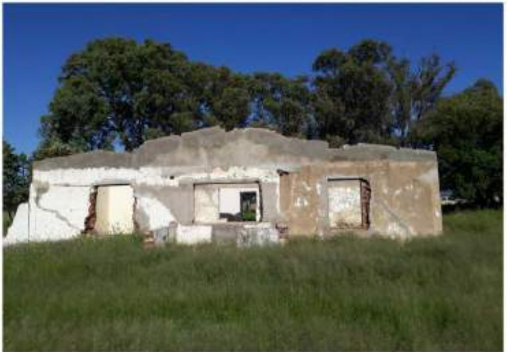
Figure 6. Western (above) and eastern (below) aspects of the main house.
