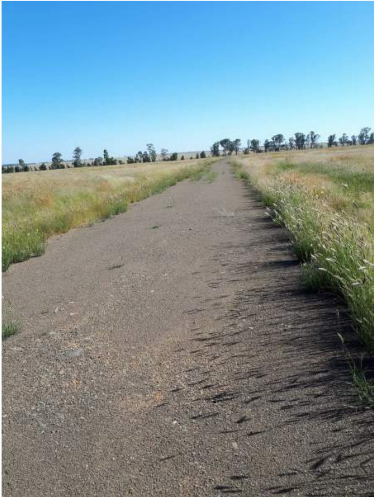
Construction of internal roads was undertaken.
