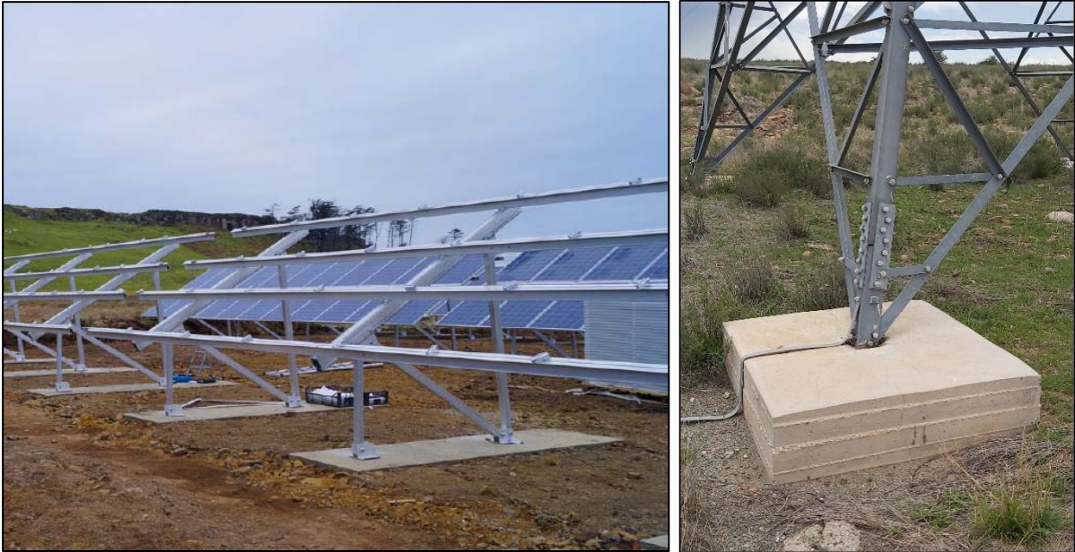
Figure 11: Typical spread (gravity) foundation systems for PV panels (left) and overhead powerlines (right)
