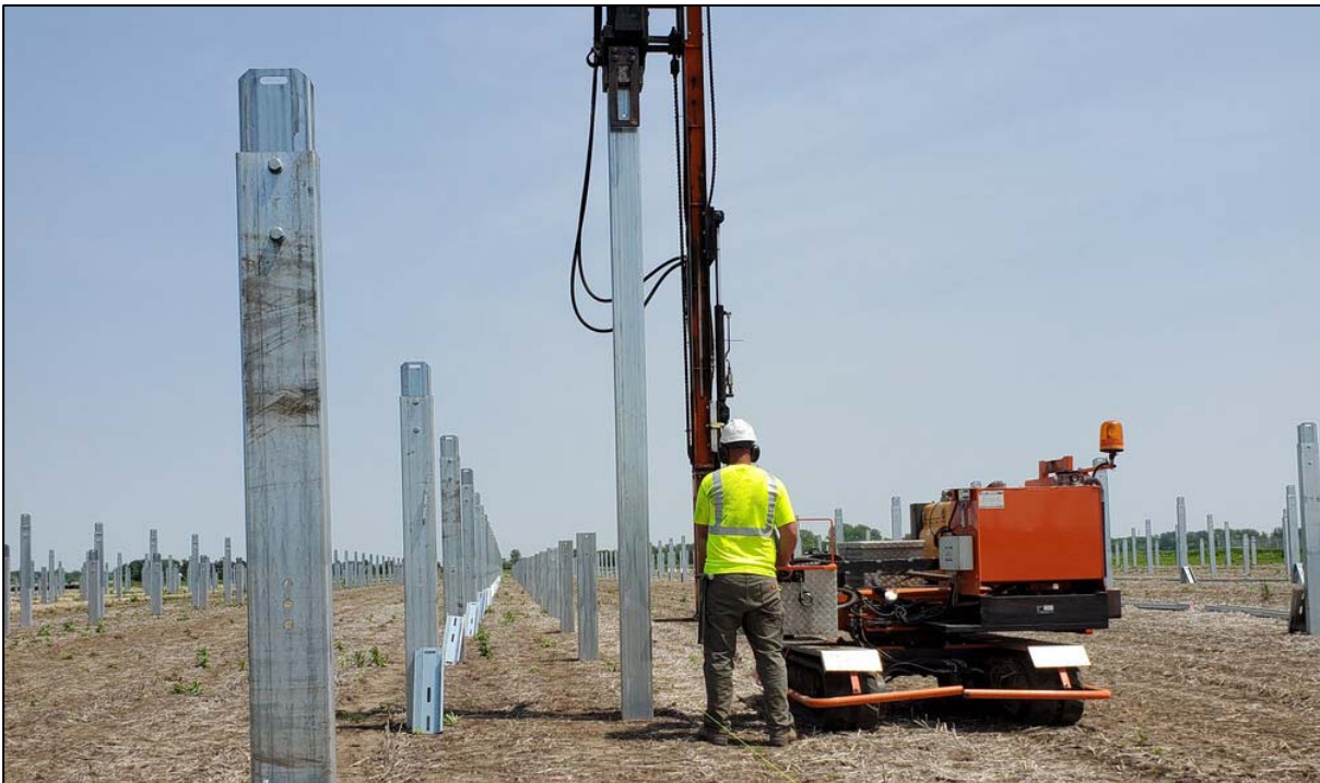
Figure 12: Driven piles for PV array frames
