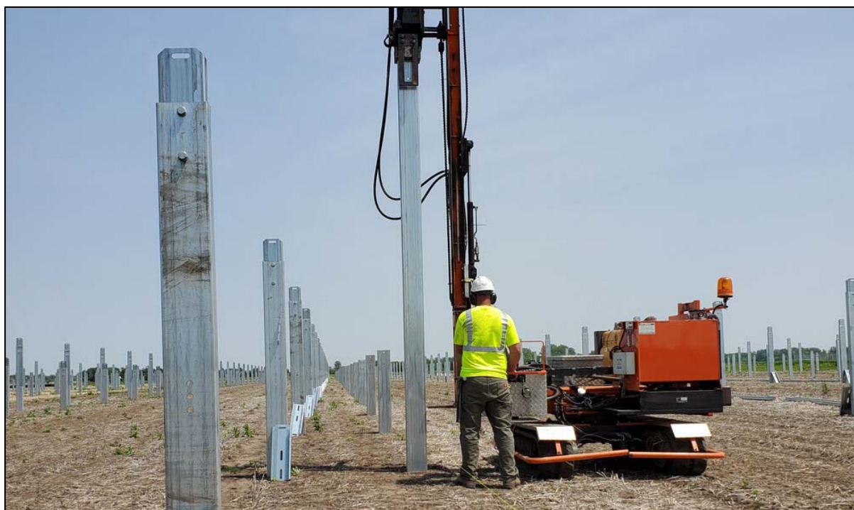
Figure 12: Driven piles for PV array frames
