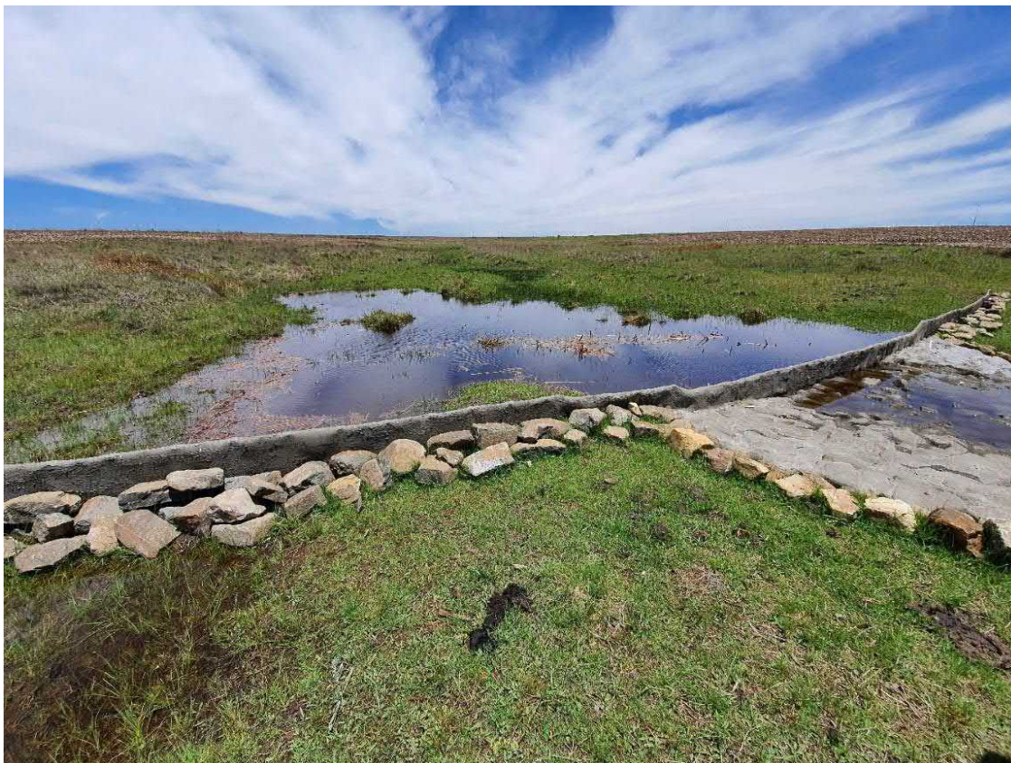
Figure 1: Typical single line Dongalock™ structure (GreenGAB, 2021)
