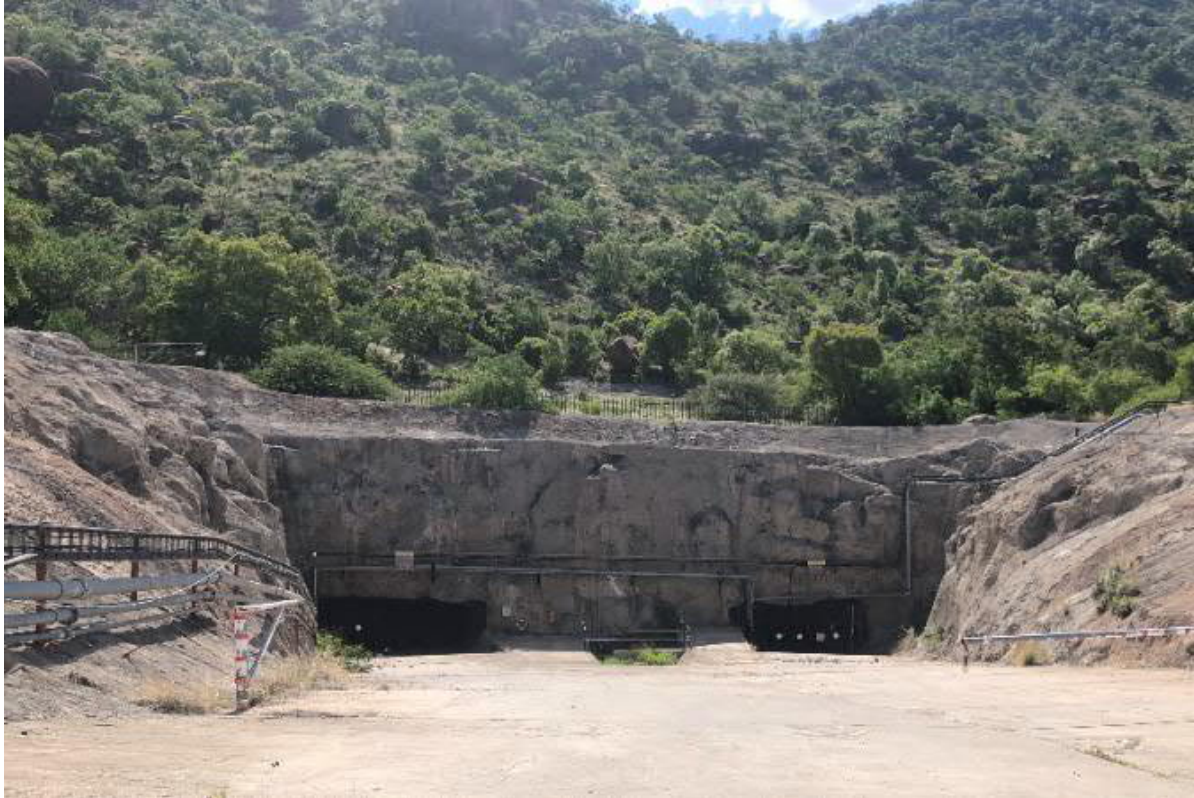
Figure 4-4: Existing Merensky Main Decline Entrance
