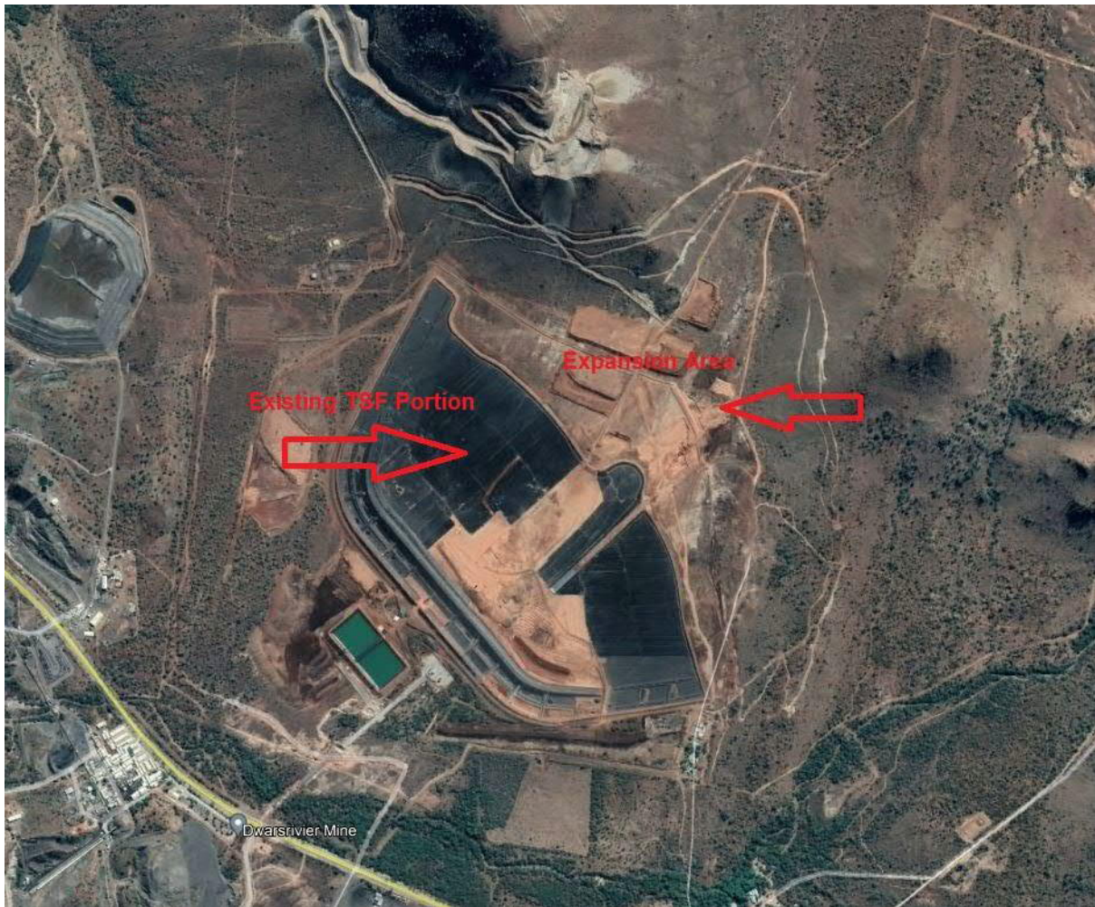
Figure 6-1: Aerial Image of TSF Expansion Area
