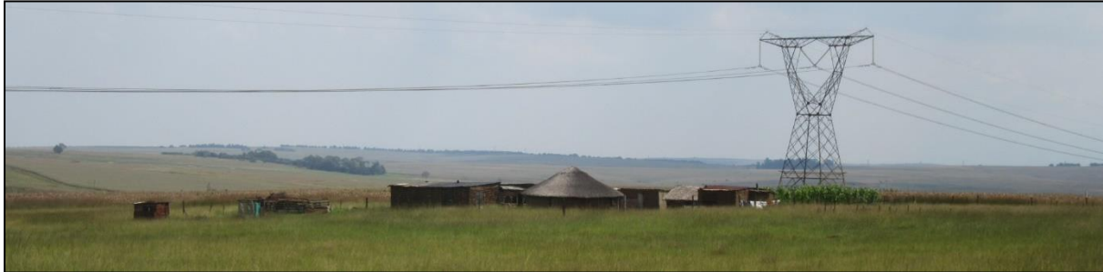
Figure 6-53: Dwellings of households with tenure rights and 400 kV line on Adrianople farm along the Overvaal Road
