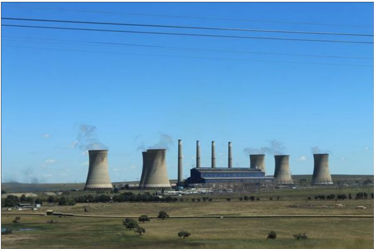
Figure 6-45: Camden Power Station
