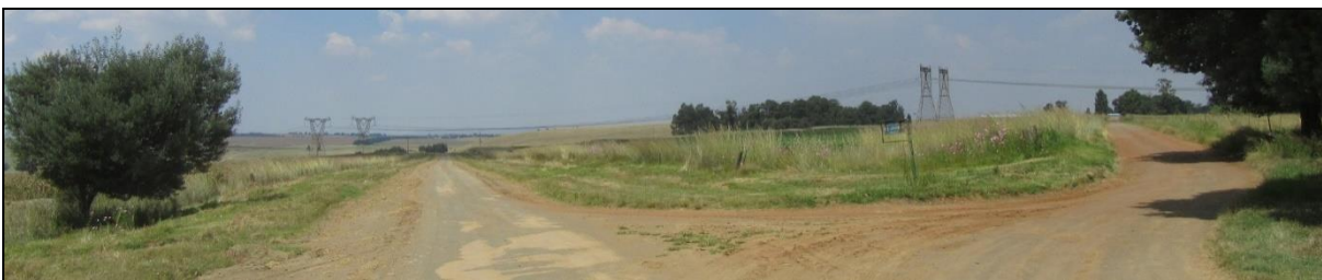
Figure 6-43: Two 400 kV lines traversing De Emigratie Road
