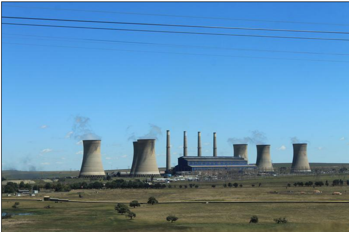
Figure 6-34: Camden Power Station
