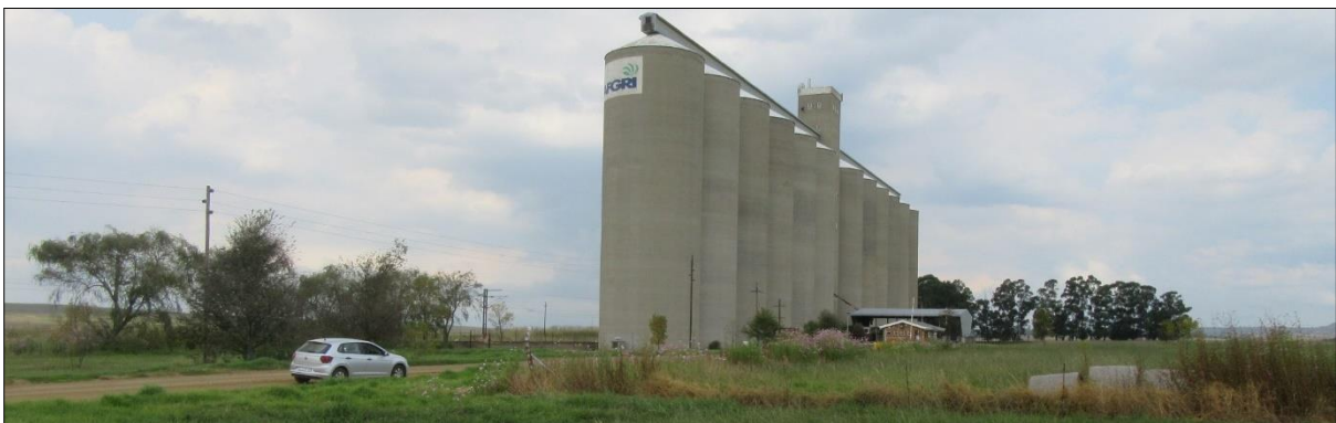
Figure 6-37: Overvaal silo located adjacent to Richards Bay railway line
