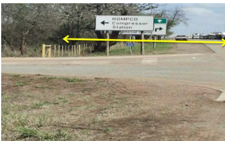
Figure 14 Proposed gas pipeline route crossing N4 road to connect to an existing Rompco pipeline
