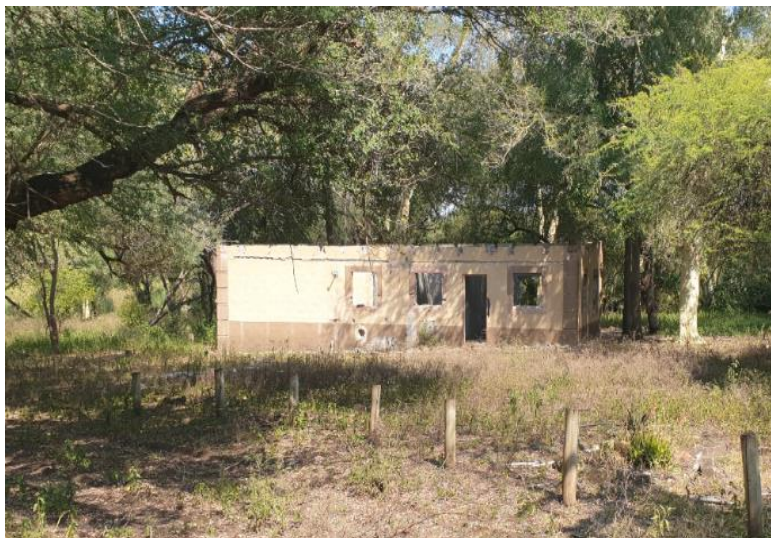
Figure 13 Abandoned Buildings on Site
