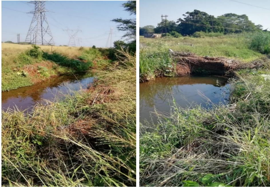
Figure 8 Drainage line running through the northern section of the site
