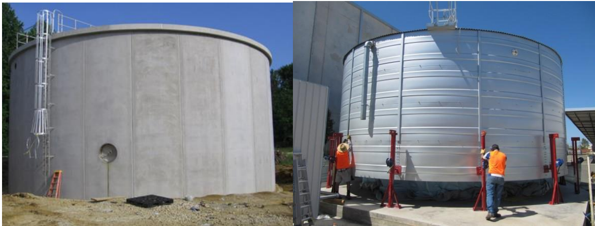
Figure 2-9: Typical water reservoir (left - concrete, right - steel)
