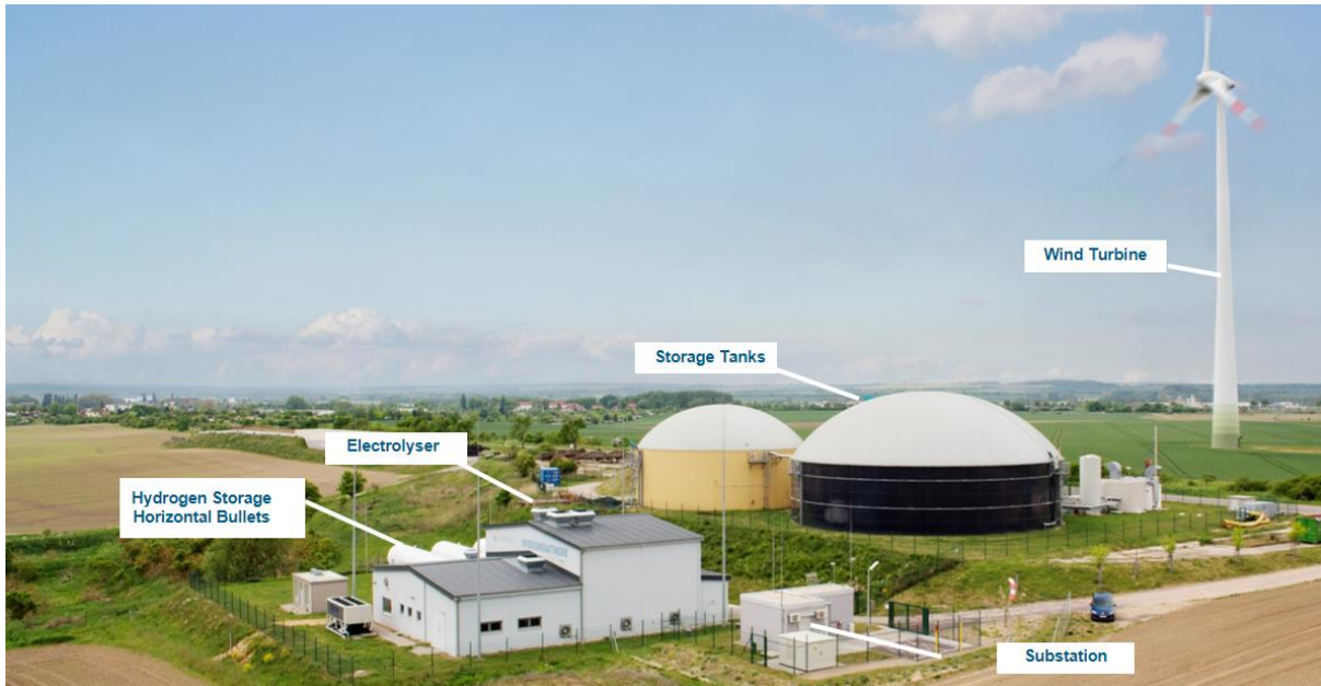
Figure 2-3: Enertrag Germany's Hybridkraftwerk
