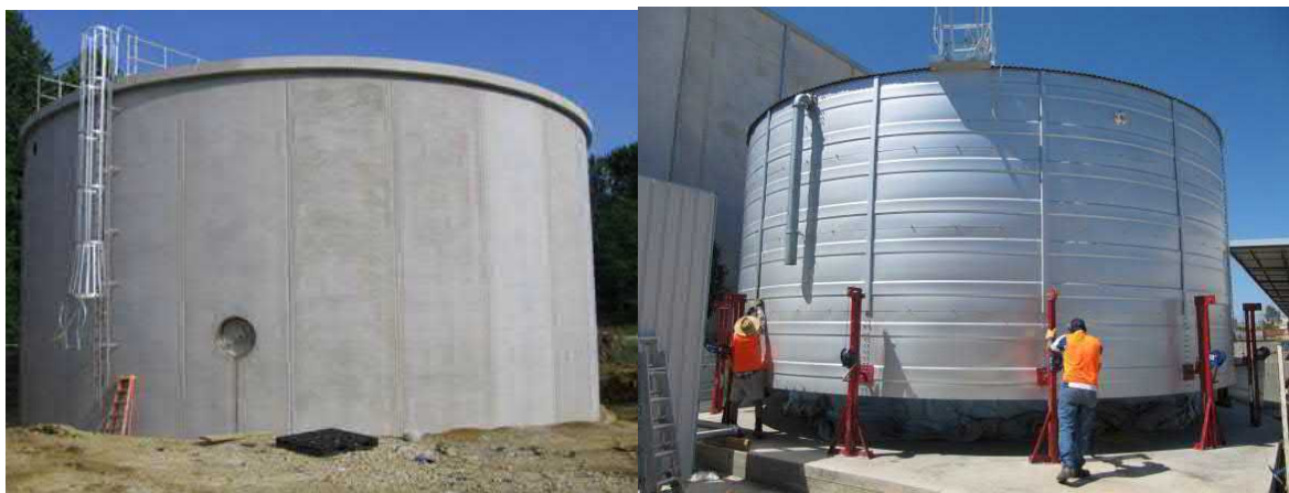
Figure 2-9: Typical water reservoir (left - concrete, right - steel)
