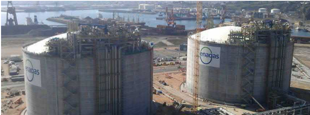
Figure 2-16: An example of a Liquid Ammonia Storage System (Source: Energas)
