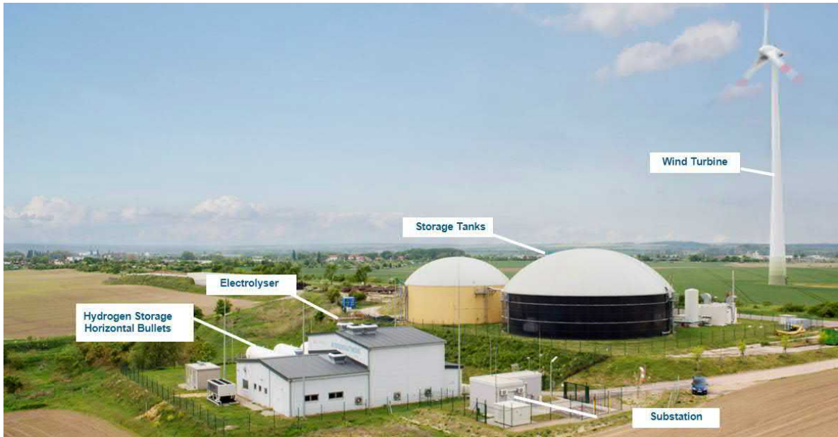
Figure 2-3: Enertrag Germany's Hybridkraftwerk
