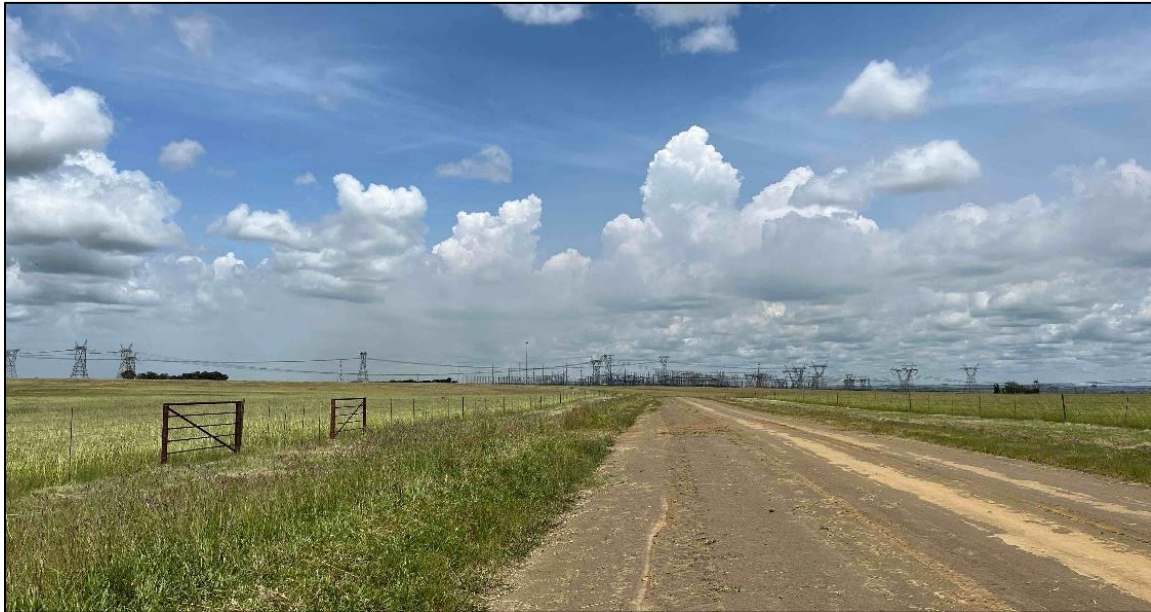
Figure 7-38: Zeus Substation south-west of the Mukondeleli WEF project area.
