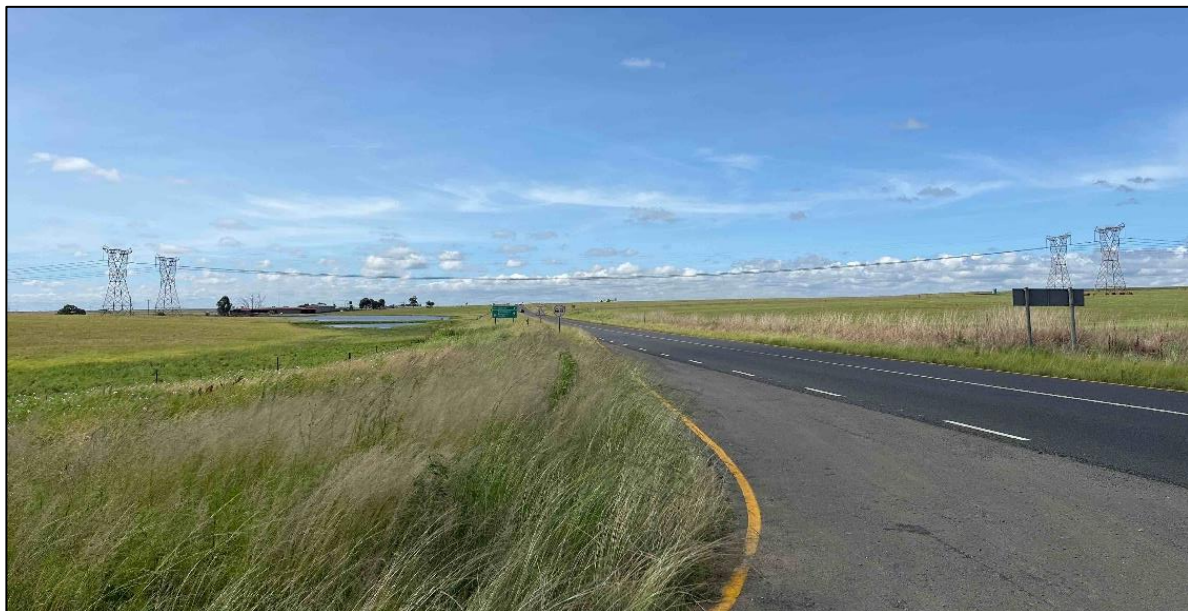
Figure 7-39: 400kV power lines High voltage power lines to the south of the Mukondeleli WEF project area
