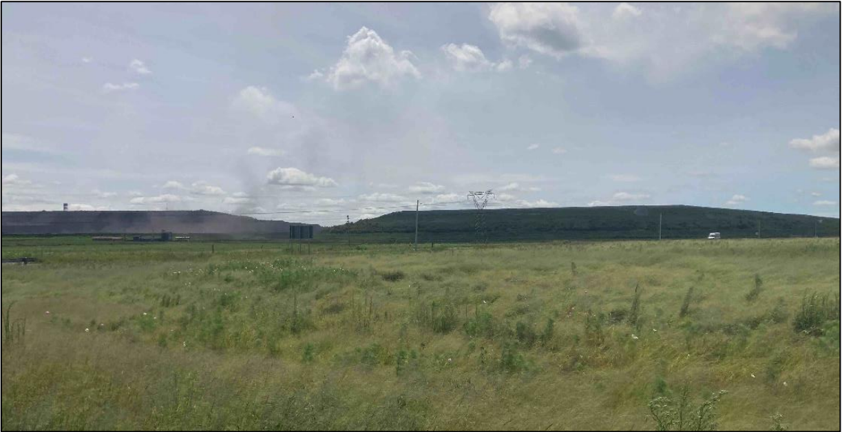
Figure 7-34: Coal dumps adjacent to the Sasol Fuel Plant
