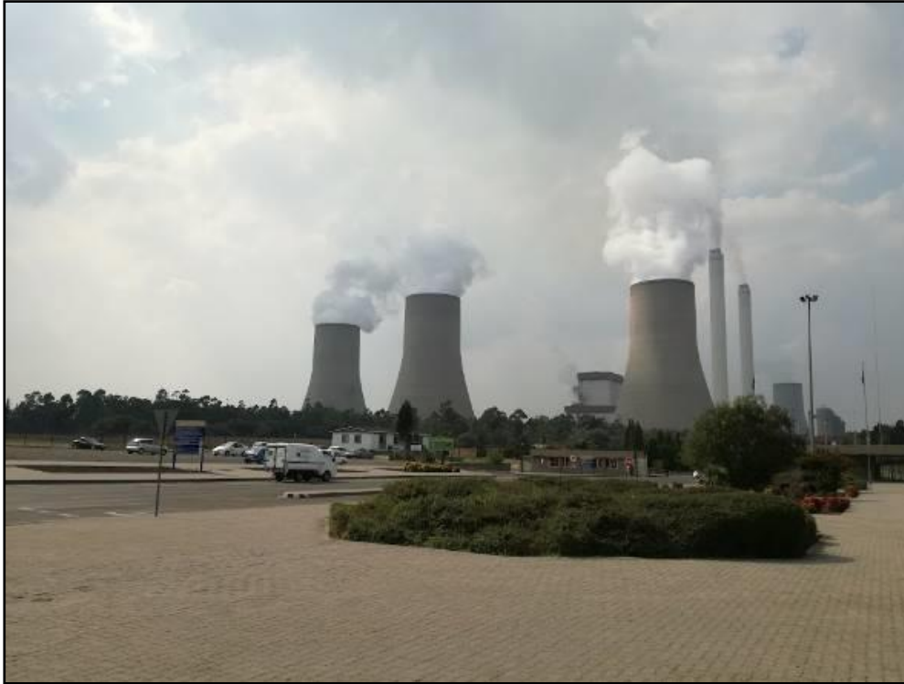
Figure 6-41 – Tukuka Power Station
