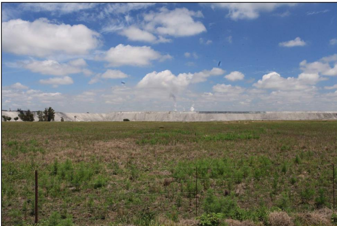
Figure 6-33 – General view of the Tourneé 2 Solar PV Park, indicating the ash dam
