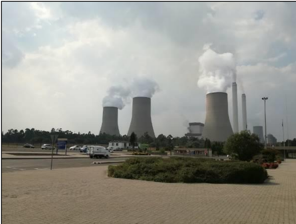
Figure 6-40 – Tukuka Power Station
