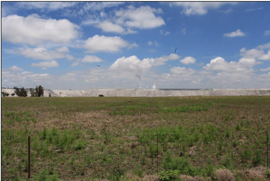
Figure 6-33 – General view of the Tourneé 2 Solar PV Park, indicating the ash dam
