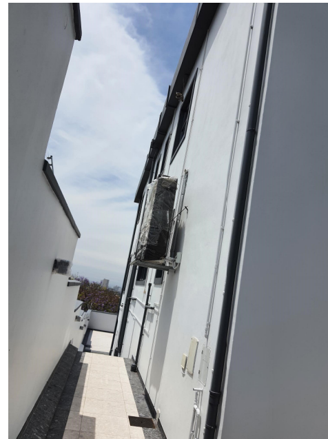
NORTH CORNER VIEWING NE ELEVATION
