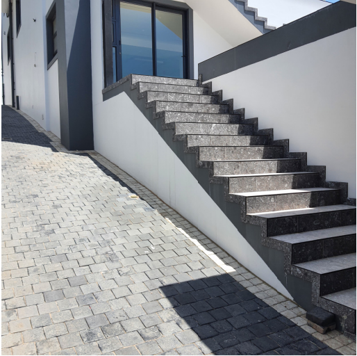
STAIRCASE DOWN TO ROAD LEVEL
