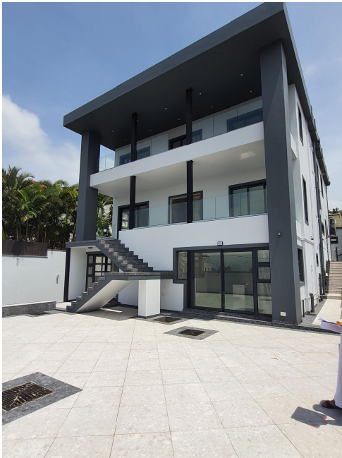
EAST CORNER VIEWING SE AND NE ELEVATIONS
