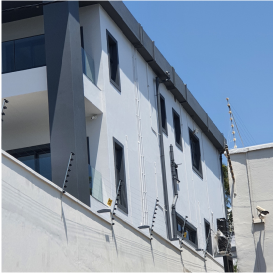
EAST CORNER FROM ROAD VIEWING NE ELEVATION
