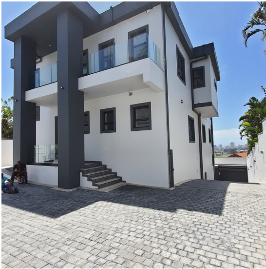
WEST CORNER VIEWING NW AND SW ELEVATIONS
