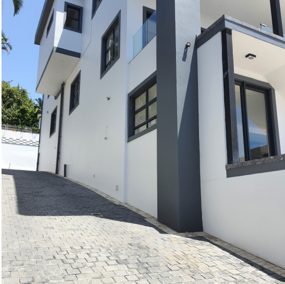
SOUTH CORNER VIEWING SW ELEVATION
