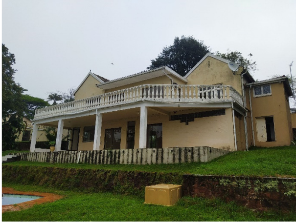
View from North East Side.
