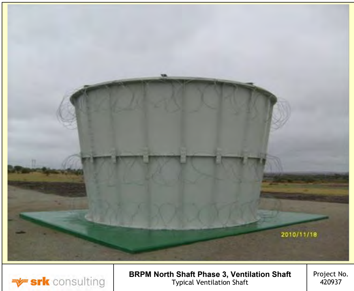
Figure 7-5: Typical Ventilation Shaft after construction
