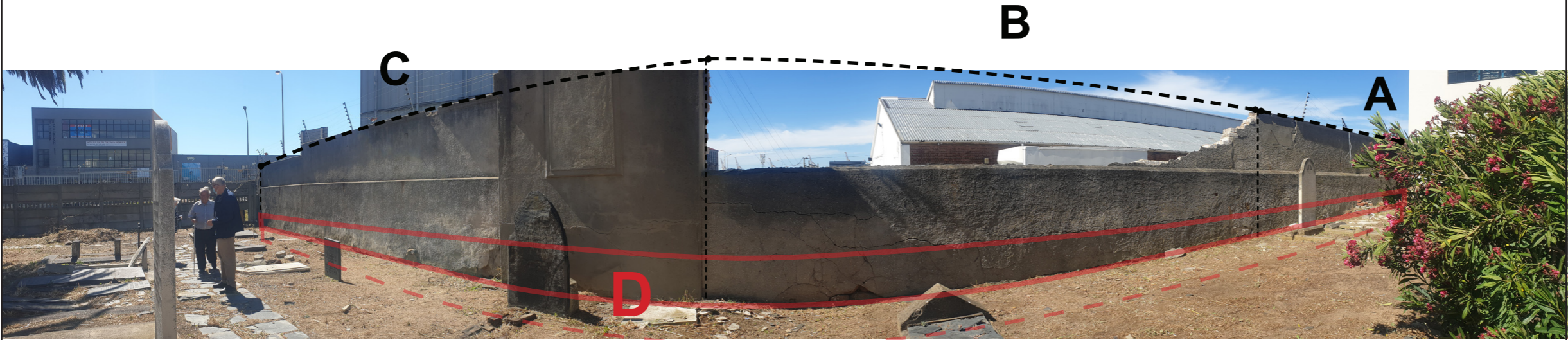
Internal photograph of the wall Indicating: Portion B which has collapsed and portions A and C which are destabilised by crumbling stone wall D.
