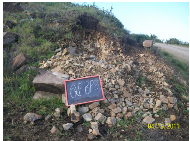
Figure C-6: QF-BP 3 showing the proximity of the road
