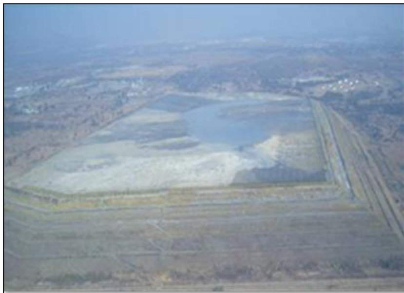
Figure 2-4: Photograph of grassed slopes of TD3, TD4 and TD5 complex
