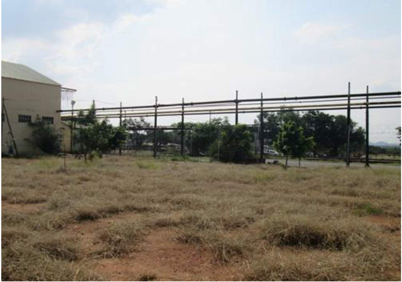
A Pipeline to the Thickener
