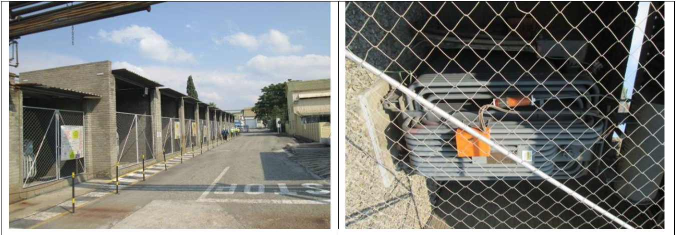
9 – Redundant Transformers: Looking in a Westerly direction from the centre of the site being demolished
