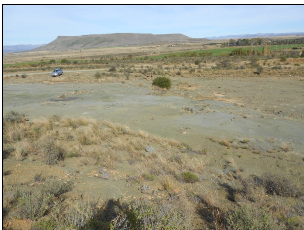
Photo C5: Poorly rehabilitated existing borrow pit 2
