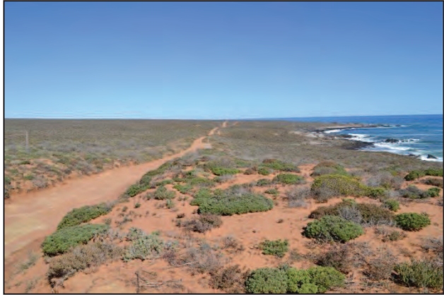
Coastal gravel road leading towards desalination plant
