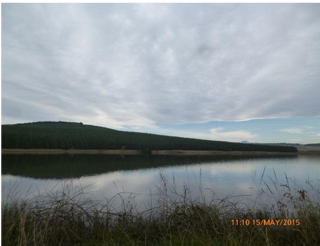
Plate 7: View of Comrie Dams East bank
