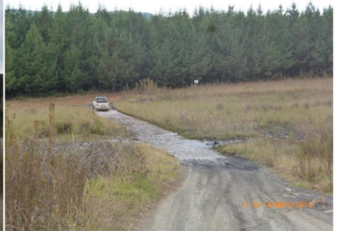
Plate 12: Existing Comrie Dam Slipway viewed from the South West bank
