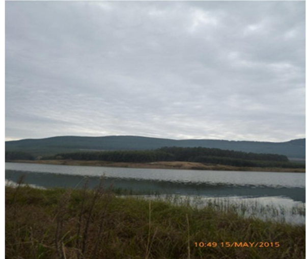
Plate 2: View of the Comrie dam from the South East bank
