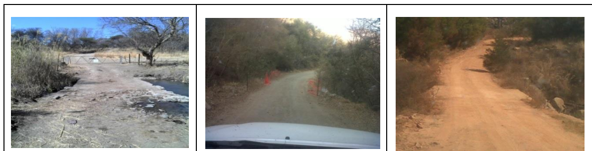
Figure 6-23: A bridge at the entrance to Richmond 370 KT, and access roads to Gamawela and Pakaneng Choma communities (SRK, 2014)
