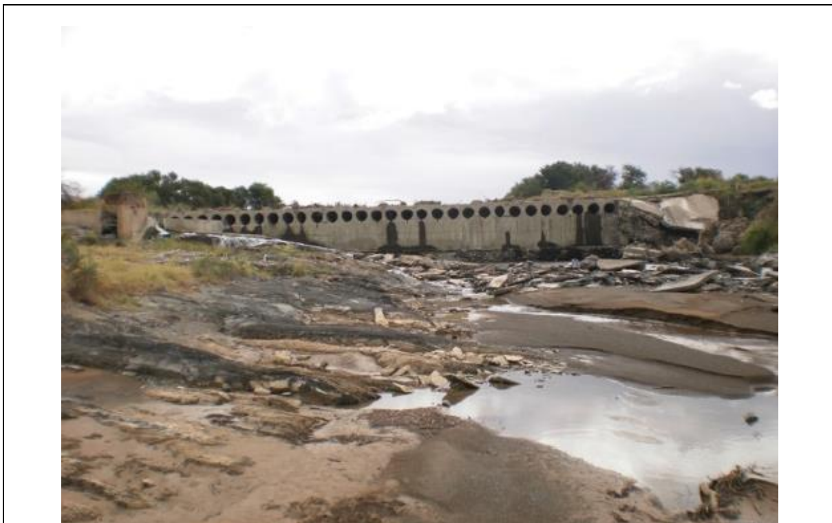
Figure 1: Crossing 10 taken from downstream.
