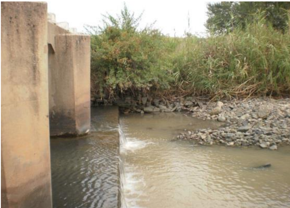
Figure 1: Crossing 6 taken from downstream.
