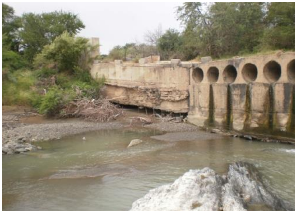
Figure 1: A view from downstream of Crossing 9.
