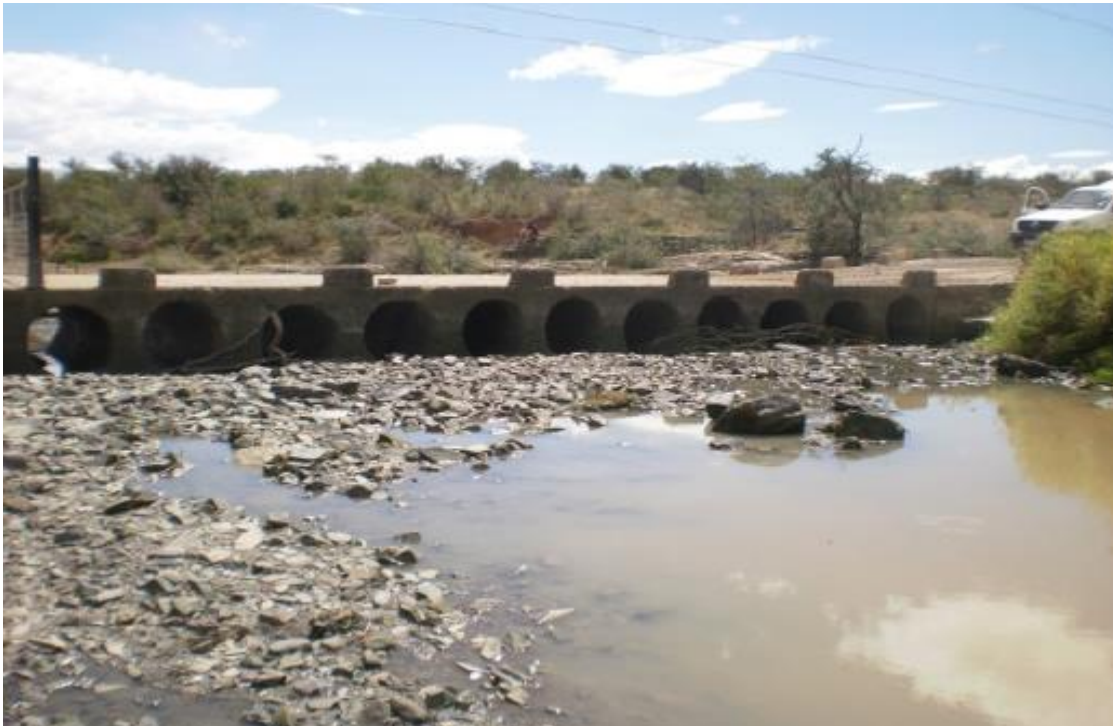
Skoenmakers River Crossing Rehabilitation Upstream view. Note gravel and boulder deposit.
