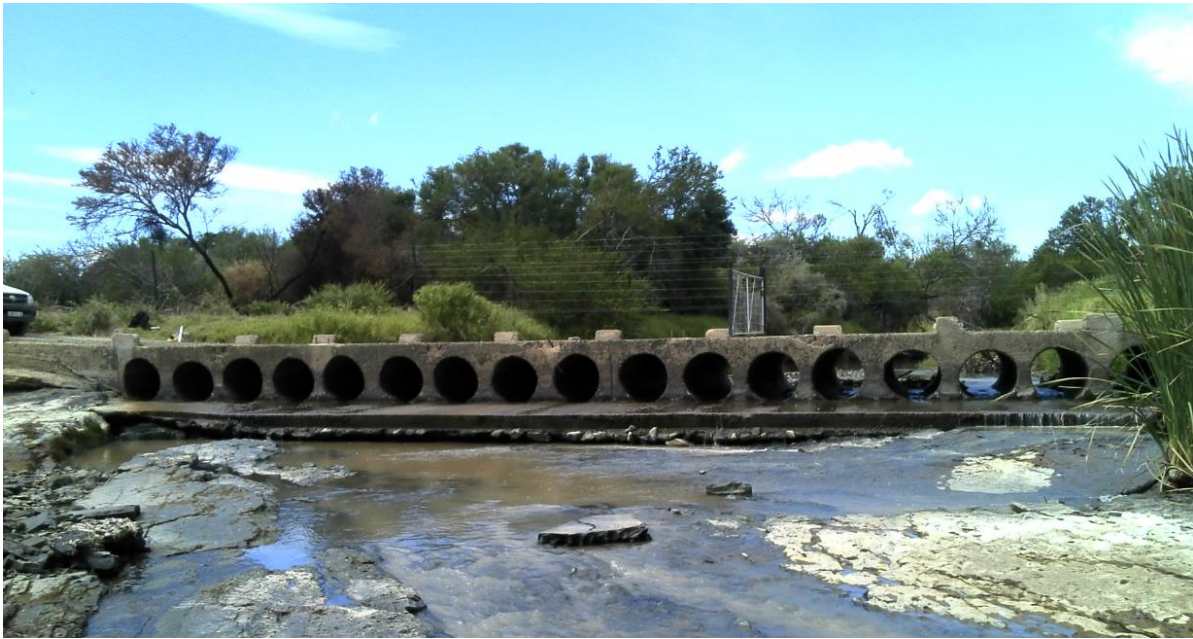
Skoenmakers River Crossing Rehabilitation Crossing 3 taken from downstream. Note the scour under the toe slab.
