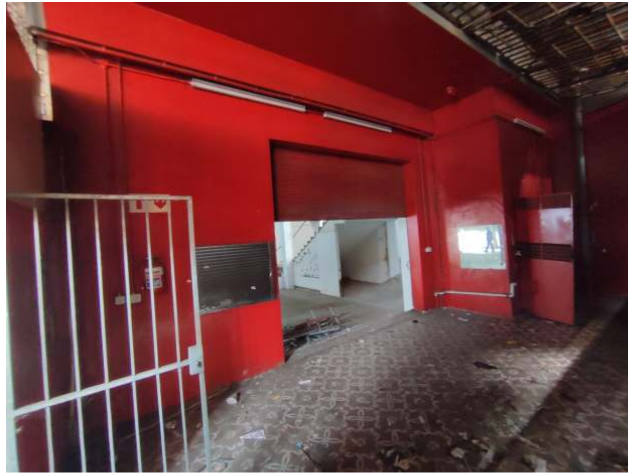
30. Existing Receiving Yard
