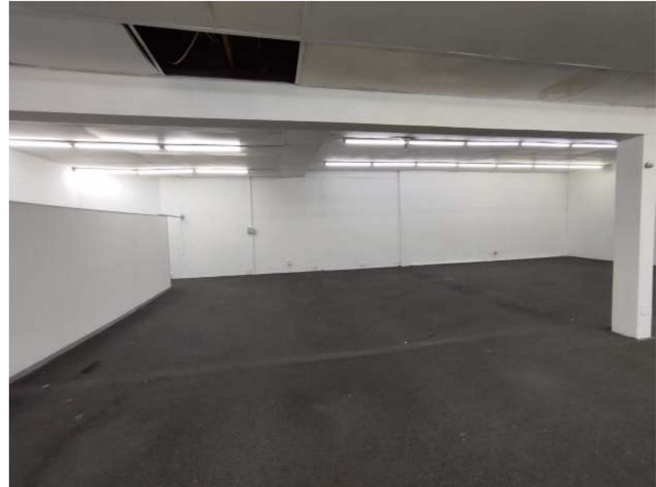
19. Existing Shop internal view
