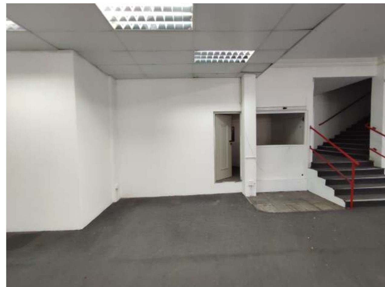
25. Existing Shop internal view - Garment Division
