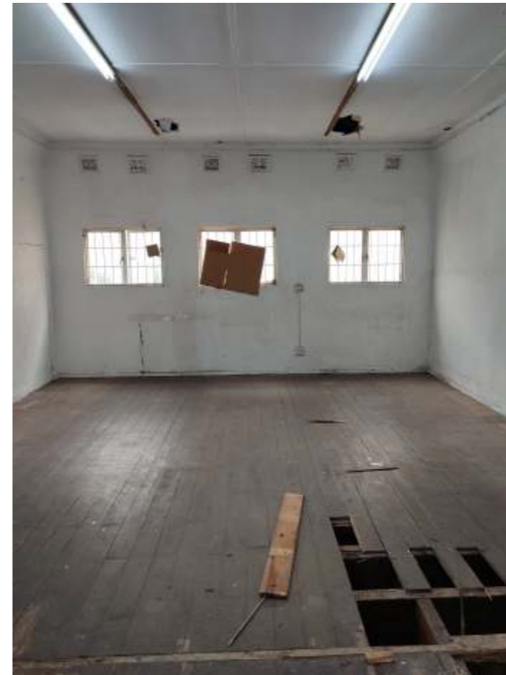
21. Existing Shop internal view
