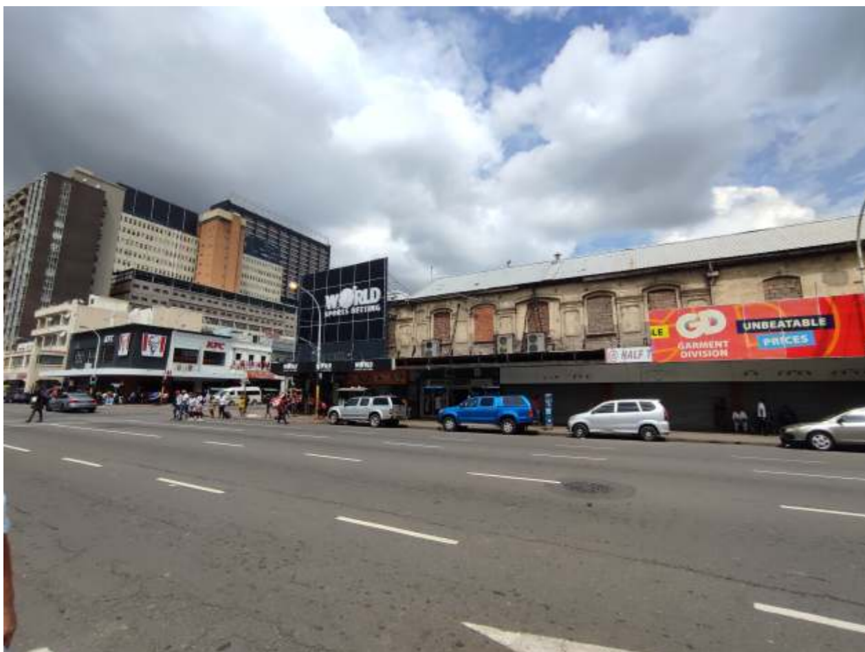
7. Portion East facade - Dr Yusuf Dadoo Street
