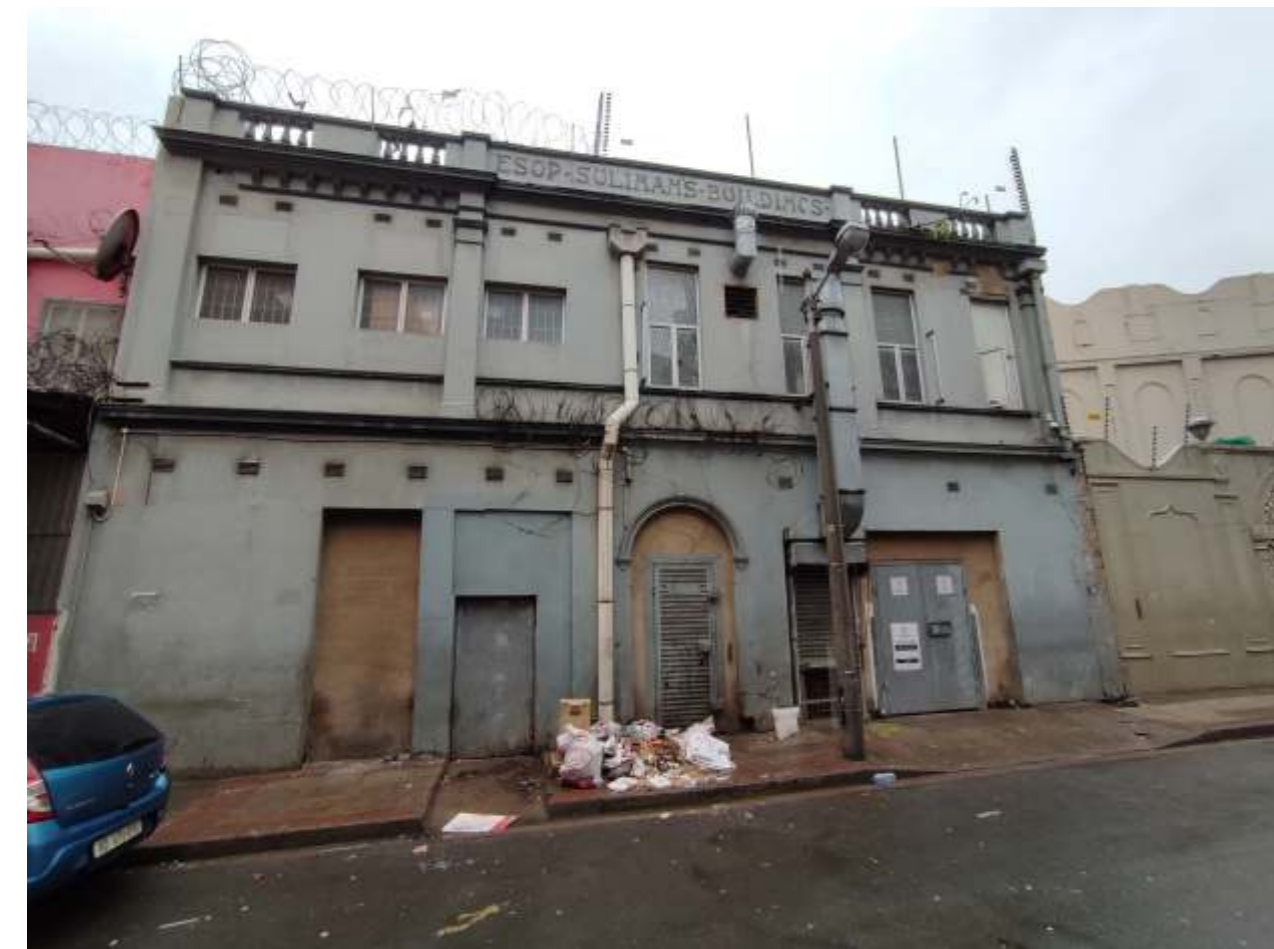
1. North Facade - Grey building on 2 Saville Street
