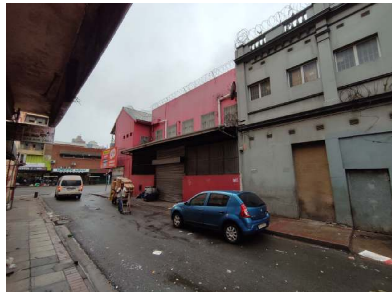
4. Looking East up Saville Street
