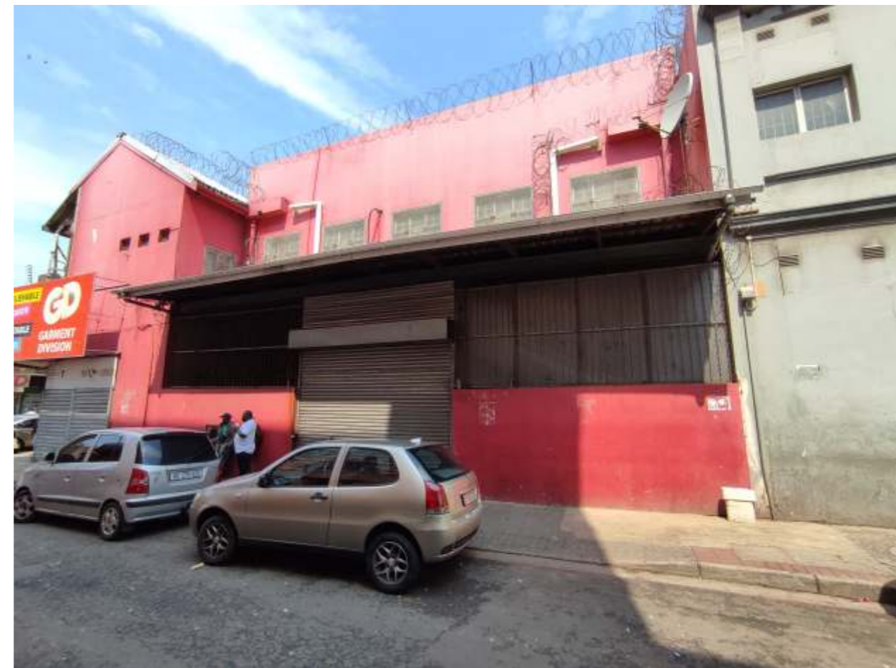
2. North Facade - Red building on 2 Saville Street
