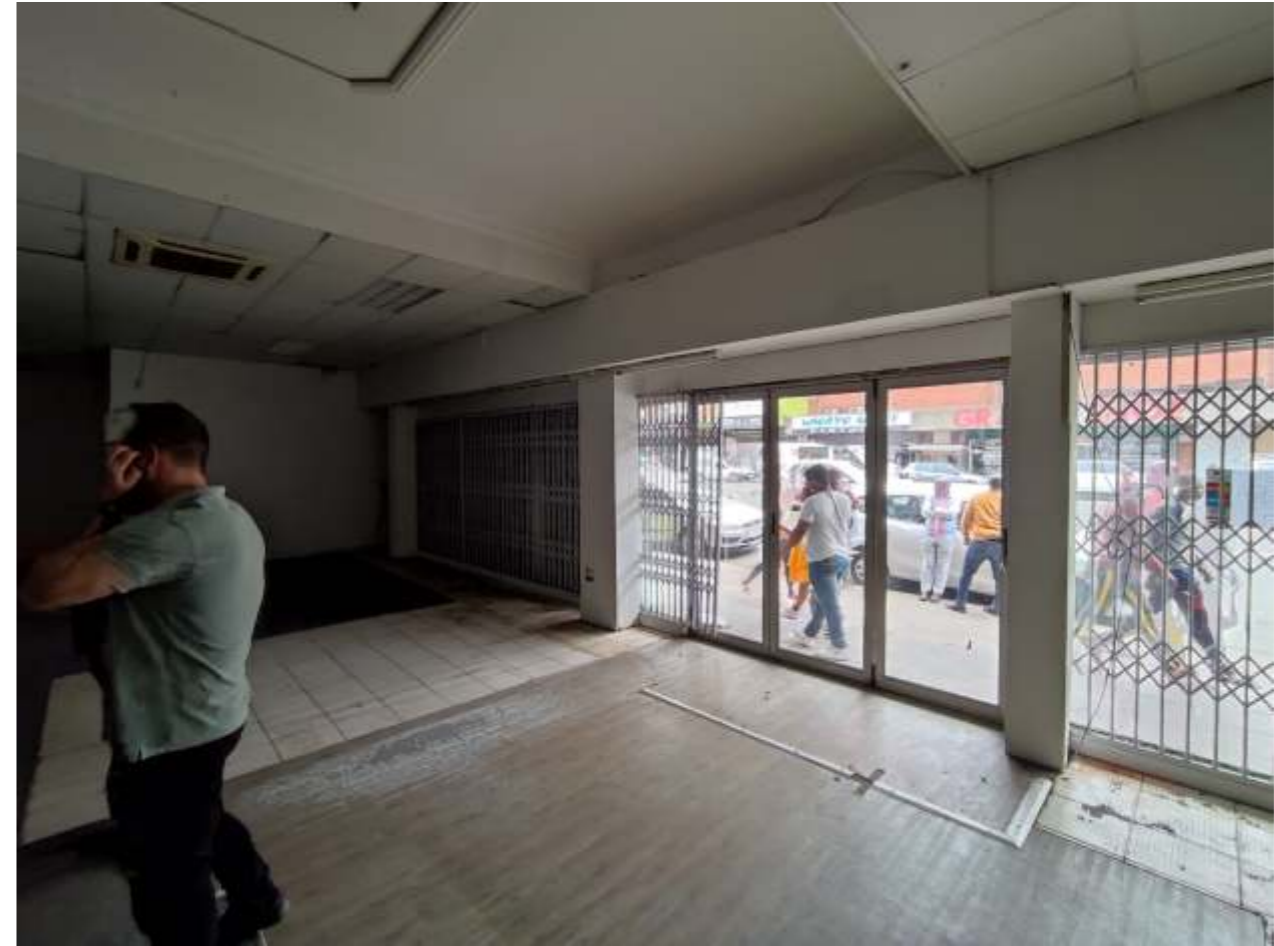
15. Existing Shop internal view
