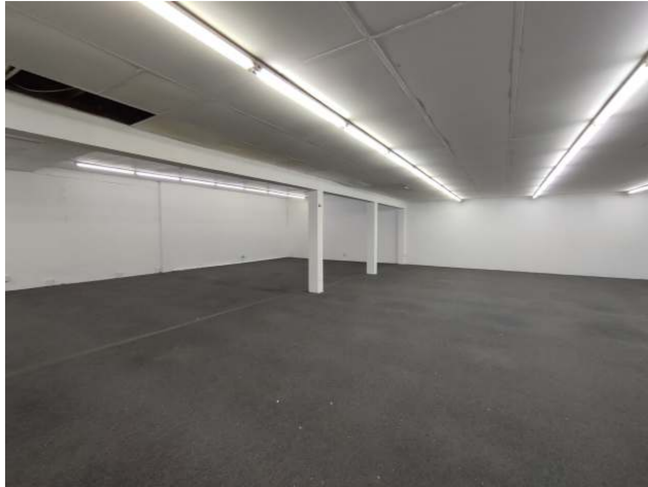
18. Existing Shop internal view
