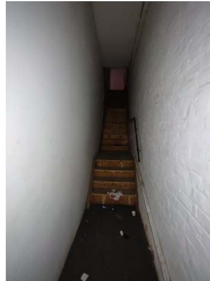
31. Existing Fire Escape from First floor
