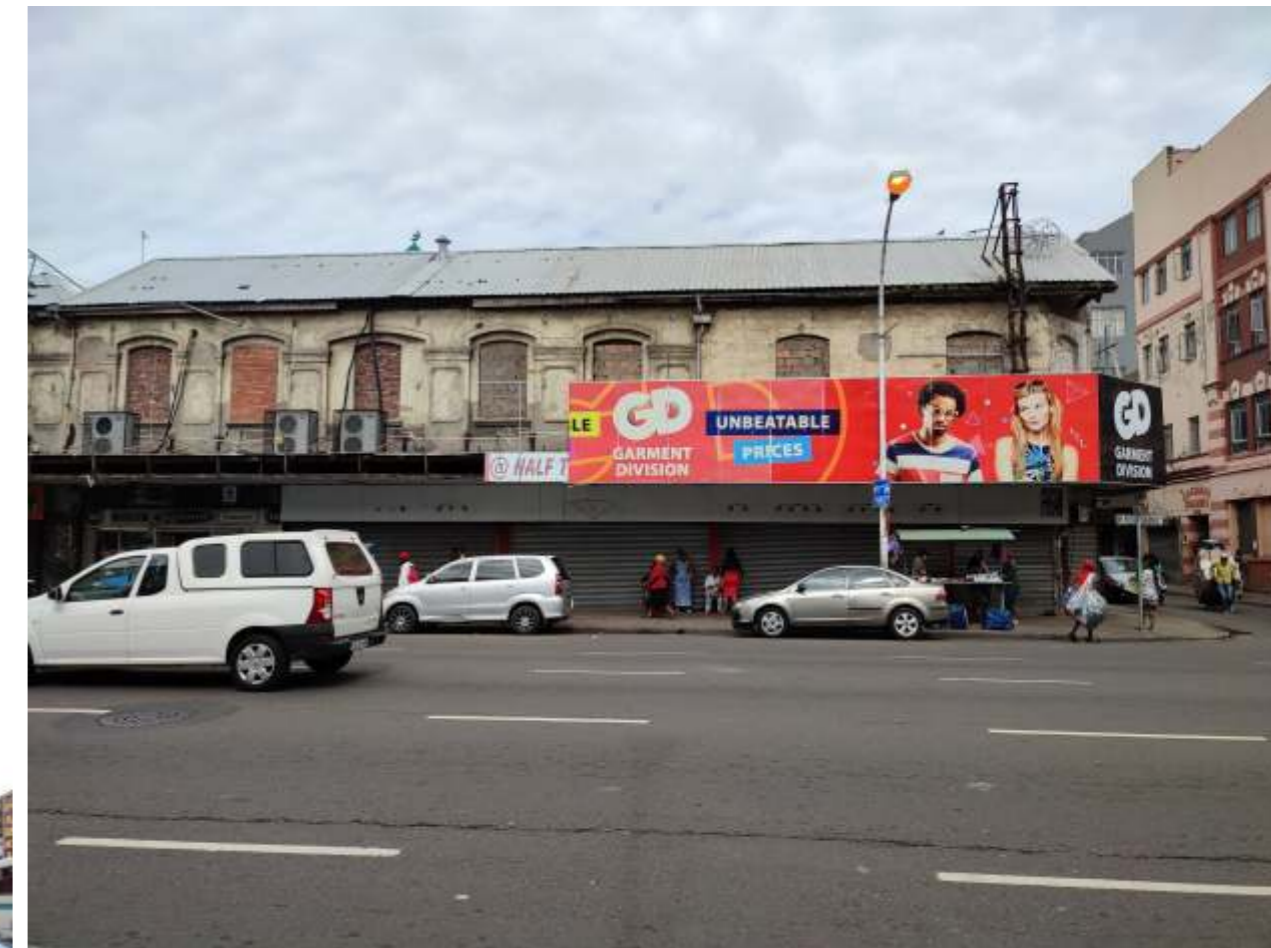
6. Portion East facade - Dr Yusuf Dadoo Street
