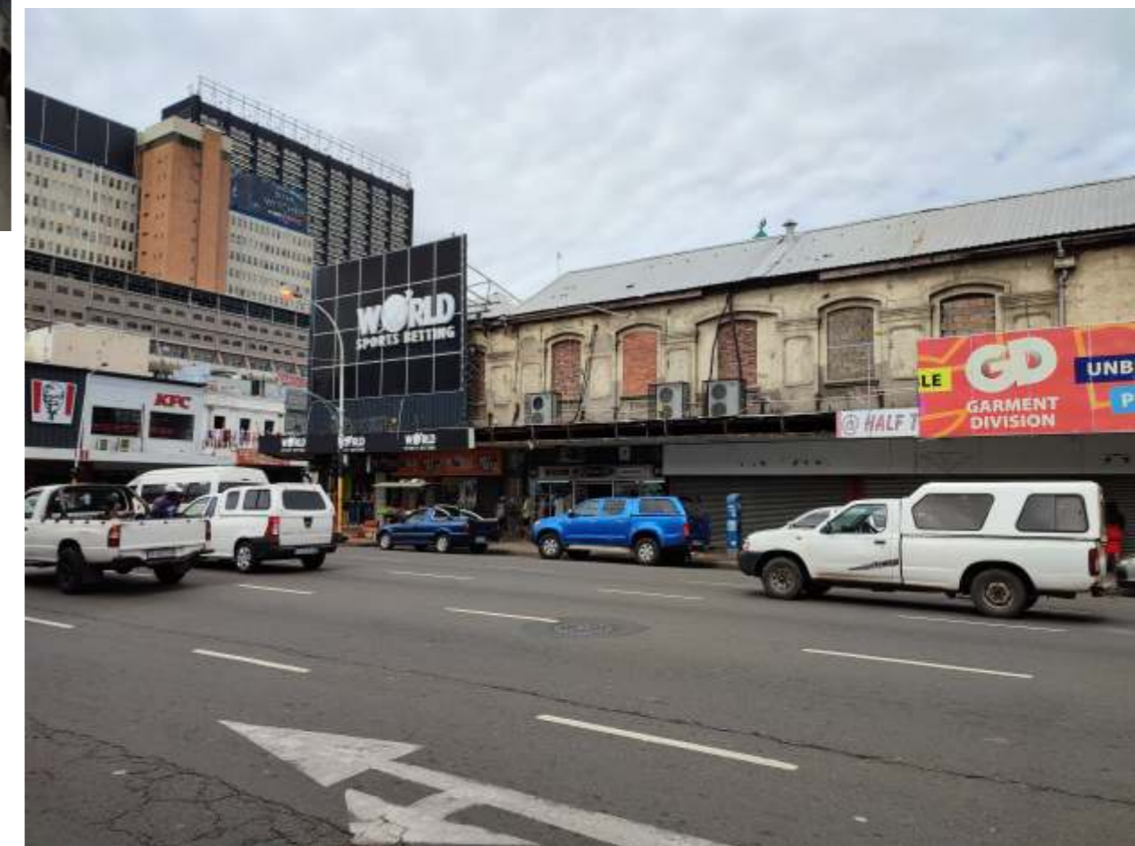
8. Portion East facade - Dr Yusuf Dadoo Street
