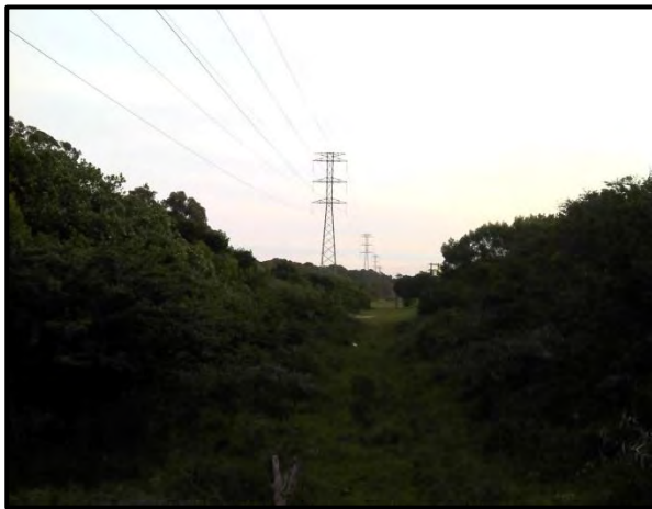
Powerline running to the south of the site parallel to Victoria drive
