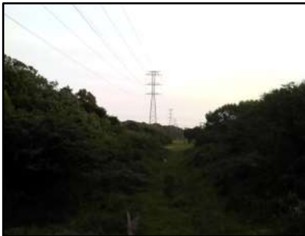
Powerline running to the south of the site parallel to Victoria drive
