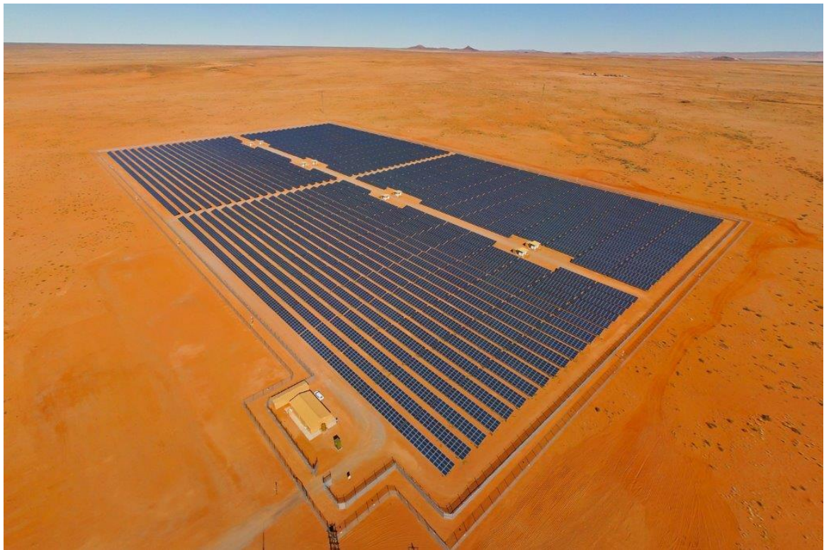
Figure 5-3: Large-Scale Photovoltaic Power Generation Facility (Source: www.pv-magazine.com )
