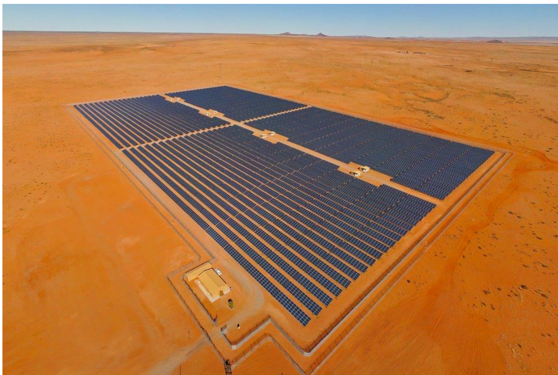
Figure 5-3: Large-Scale Photovoltaic Power Generation Facility (Source: BioTherm)
