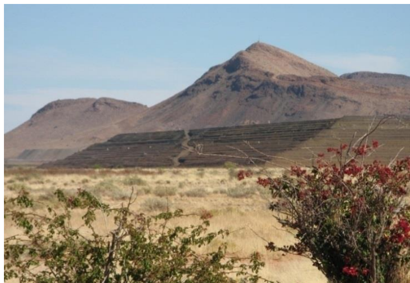
Figure 6-12: Black Mountain Tailings Dam
