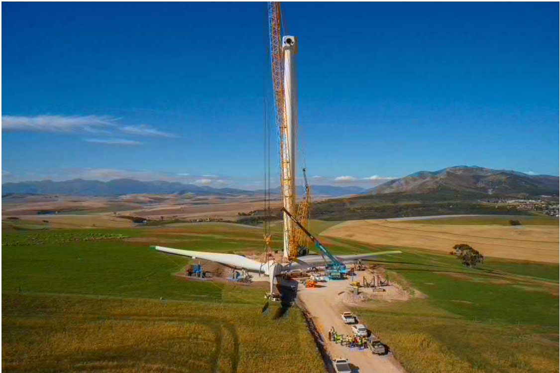
Figure 7-2: Construction of the Turbine – Preparing to lift the Rotor
