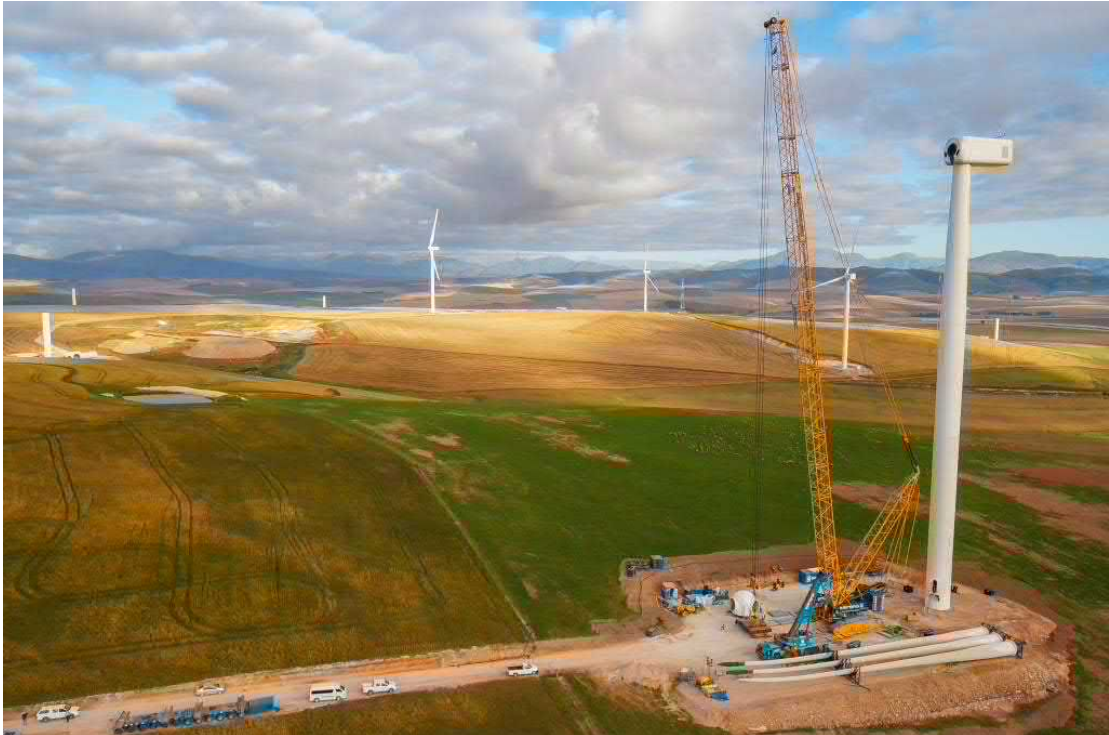
Figure 7-3: Construction of the Turbine – Lifting Equipment (i.e. Crane)
