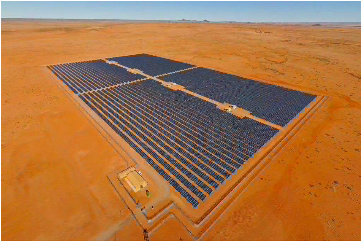
Figure 7-1: Large-Scale Photovoltaic Power Generation Facility (Source: BioTherm)
