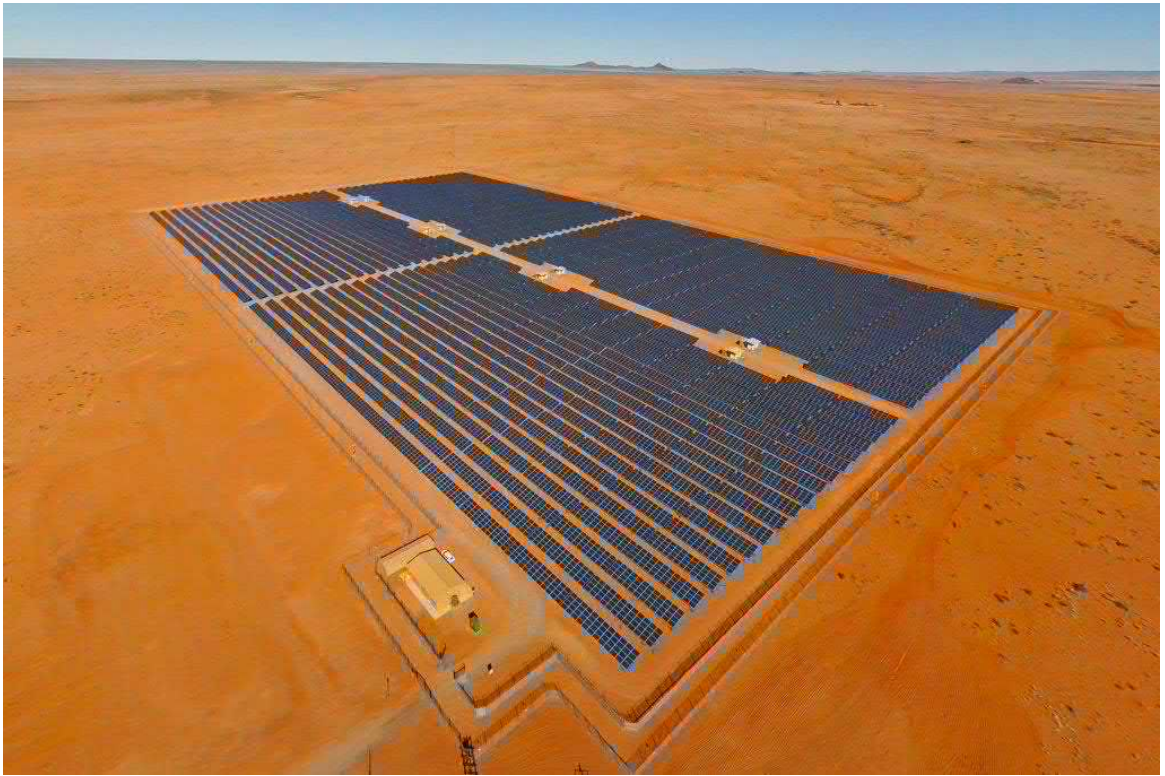
Figure 7-1: Large-Scale Photovoltaic Power Generation Facility (Source: BioTherm)
