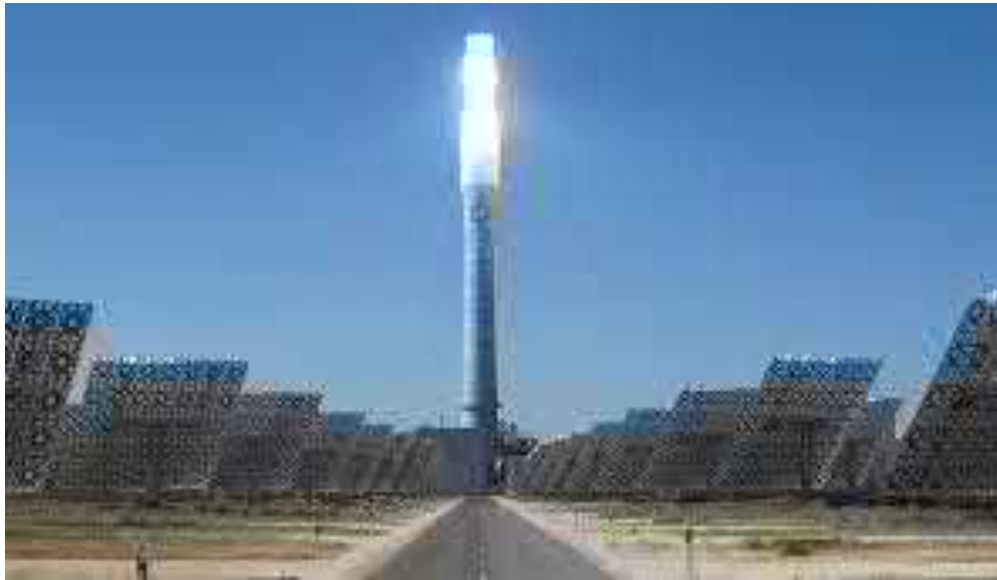
Figure 7-8: Central Receiver (Source: www.torresolarenergy.com )
