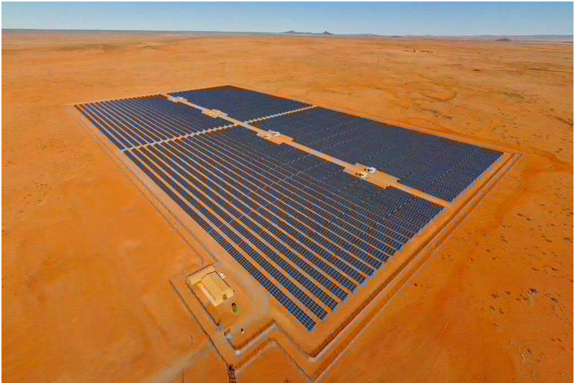
Figure 7-1: Large-Scale Photovoltaic Power Generation Facility (Source: BioTherm)
