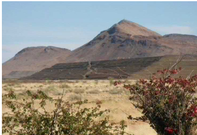
Figure 8-13: Black Mountain Tailings Dam
