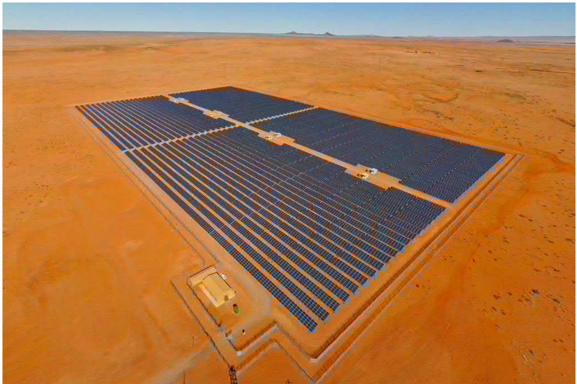
Figure 7-1: Large-Scale Photovoltaic Power Generation Facility (Source: BioTherm)
