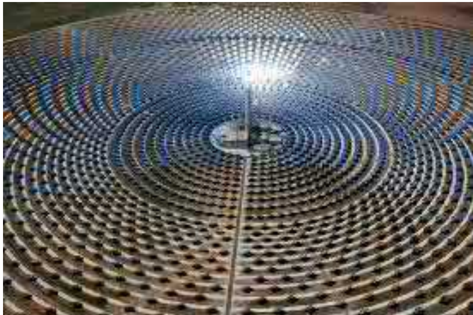
Figure 7-9: Elliptical formation of the Central Tower Solar Field (Source: www.finetubes.co.uk )
