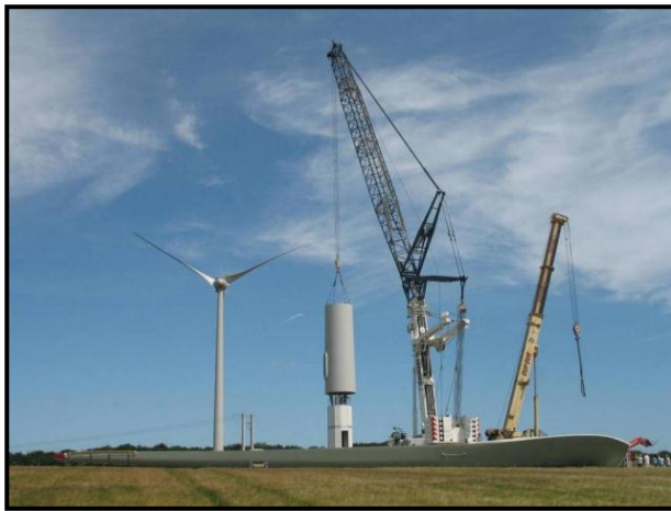
Figure 2-7: Assembly and erection of the tower sections using cranes
