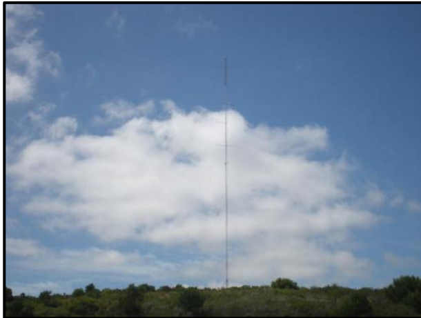
Figure 2-3: An example of a meteorological mast (CES, 2014)
