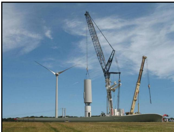
Figure 2-6: Assembly and erection of the tower sections using cranes (CES, 2014)
