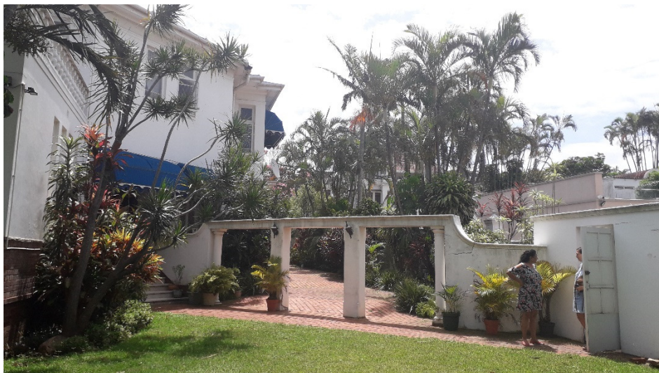
East elevation and entrance from Overdale Rd
