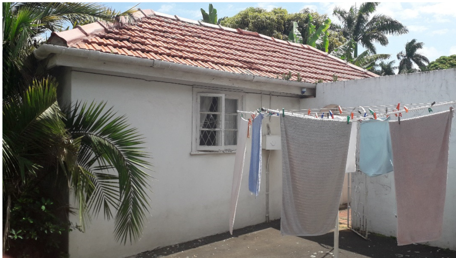
Outbuildings on the West boundary (shared with 3 Overdale Rd)
