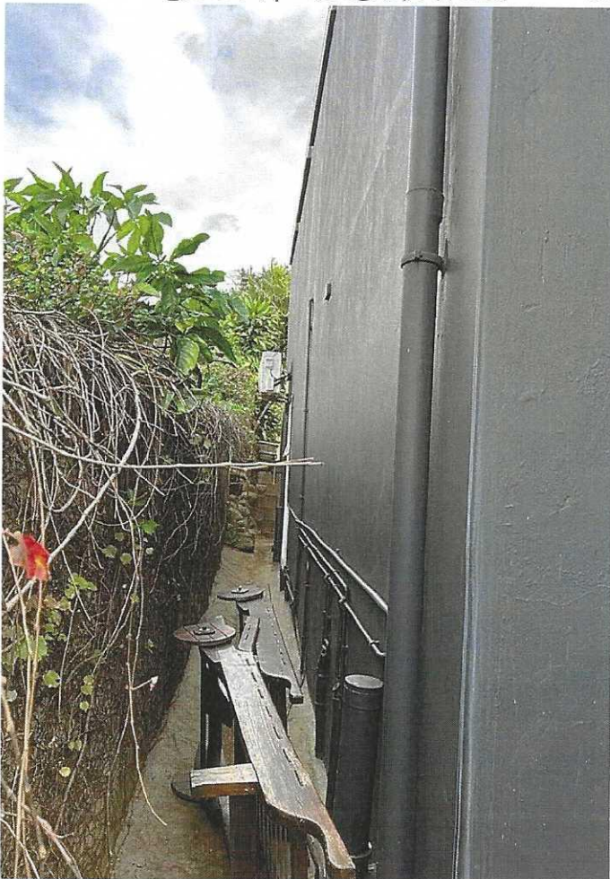
(Difficult to photograph) SOUTH ELEVATION - outbuilding
