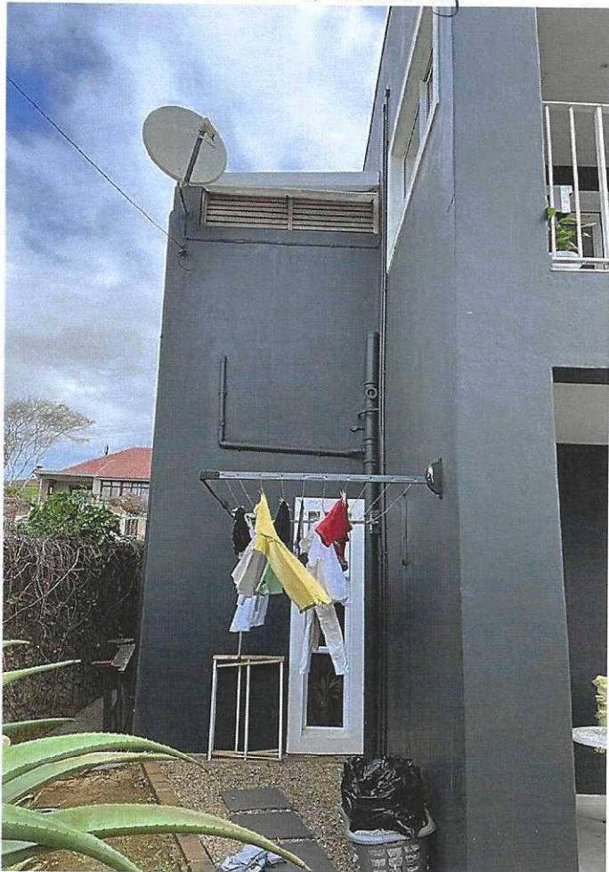
East Elevation - outbuilding
