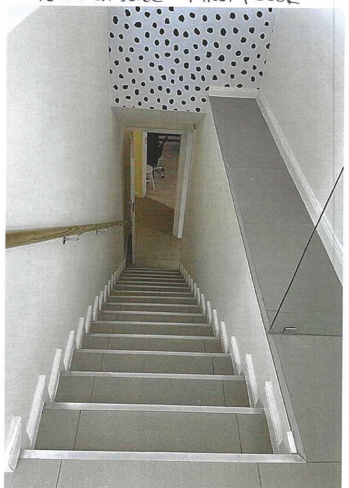
NEW STAIRS - main dwelling
