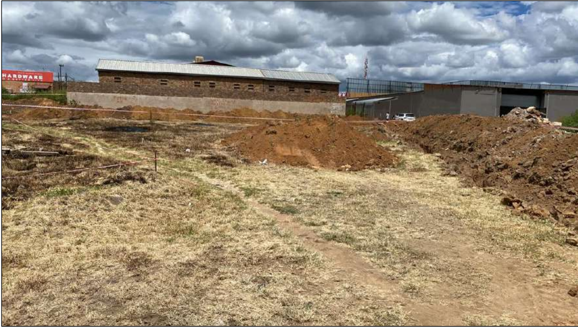
Figure 7 – Trenches being dug for the water diversion.
