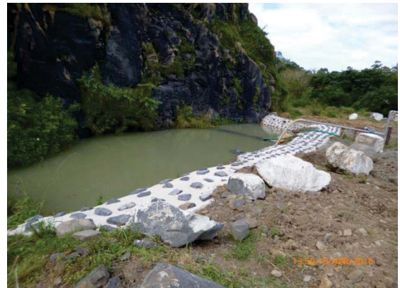
Plate 20: Final Settlement Pond, water abstracted for dust suppression.
