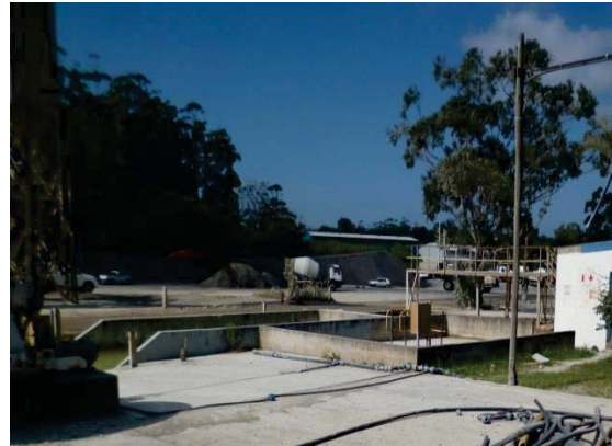
Plate 14: Cement water settlement facility
