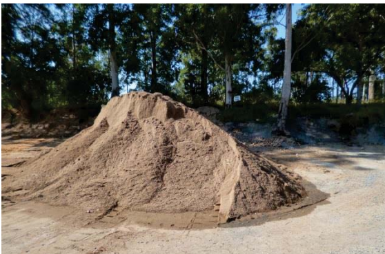
Plate 5: Sand Stockpile for use in concrete batch plant.
