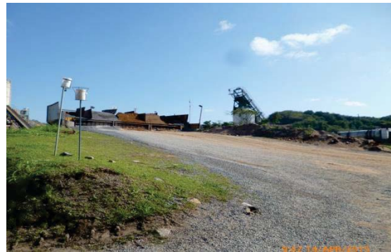
Plate 8: Ramp Up to Cold feed bins of Concrete Batch Plant.
