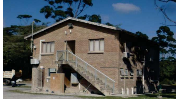
Plate 2: Weigh Bridge offices.
