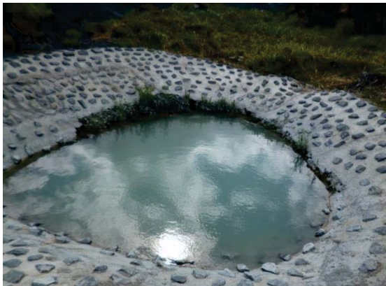
Plate 19: 2nd Settlement Pond, overflows to 3rd settlement pond (final settlement pond)
