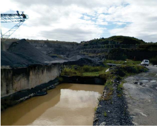
Plate 23: Initial settlement of sediments in existing Channel C8.1 .
