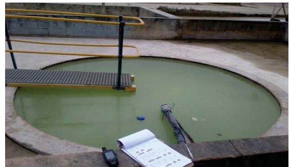
Plate 23: Concrete Pond, containment of water from the Concrete Batch Plant
