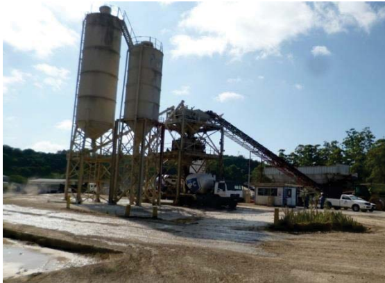
Plate 13: Concrete Batch Plant area.
