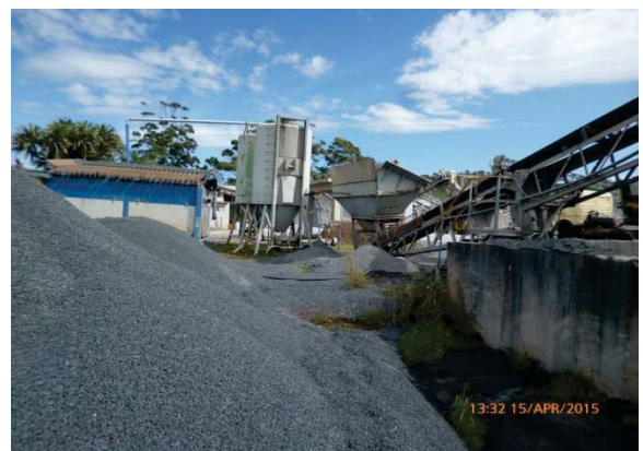
Plate 22: Wash Plant Facility with washed aggregate stockpiles.
