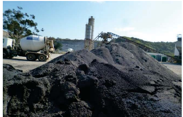
Plate 4: Reclaimed Asphalt Gravel, with no bunding.
