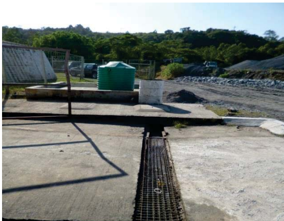
Plate 17: Cut off trench reporting to the Oil Trap system
