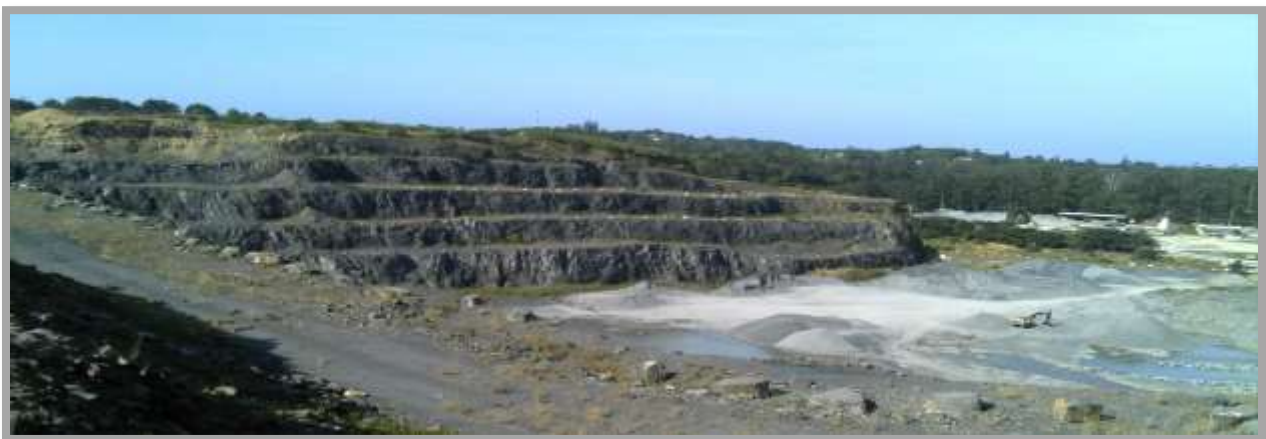
FIGURE 1 EXISTING SCSC DWYKA TILLITE QUARRY
