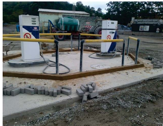
Plate 18: Filling Station on hardstanding and bunding in place.
