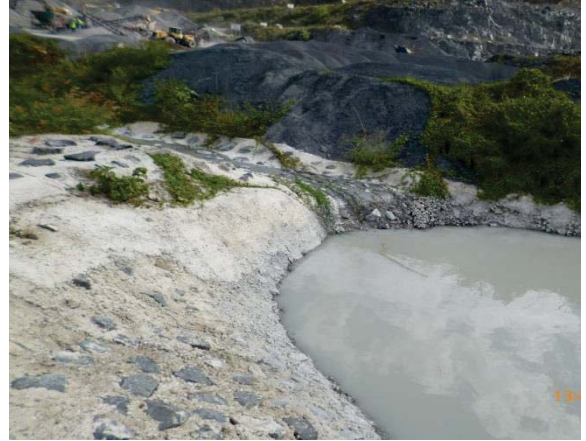
Plate 24: Runoff from channel C8.2 reporting to the 1 st settlement pond .
