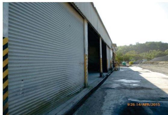
Plate 16 : Cut off trench outside the workshop
