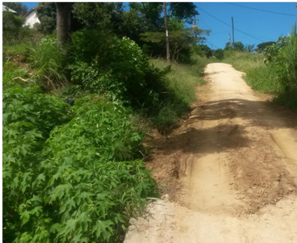
Figure 6: Vegetation around the existing culvert
