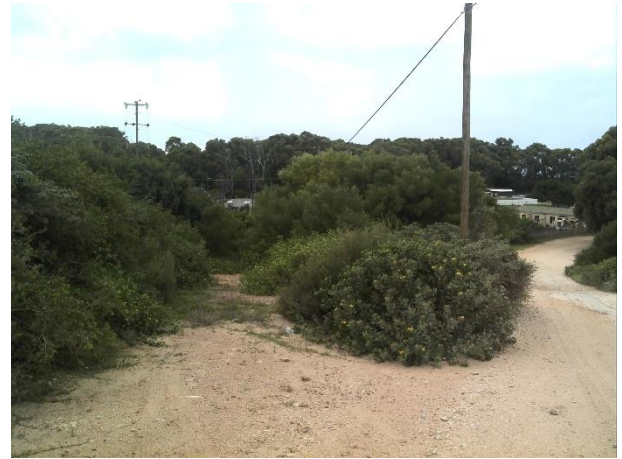
GM2-1: Gravel road behind the Seaview pump station complex to the north east. On the option 2 pipeline alignment Photo 36
