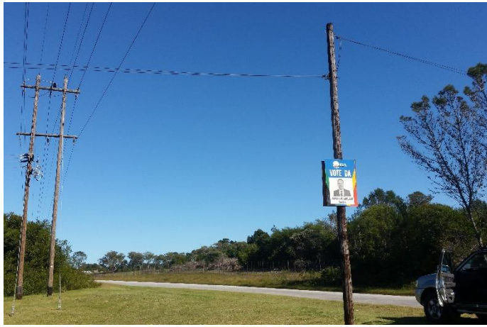
13g: Telephone pole within the road reserve Photo 19
