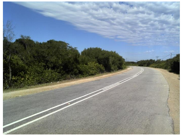
GM1-3: Option 1 pipeline alignment adjacent to the Seaview Rd Photo 42
