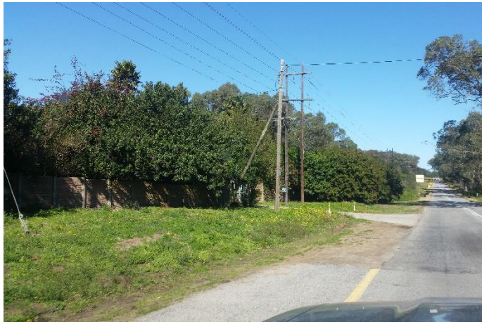
8g: Some landowner driveways will be crossed by the Greenbushes pipeline alignment. Note the powerline. Photo 13
