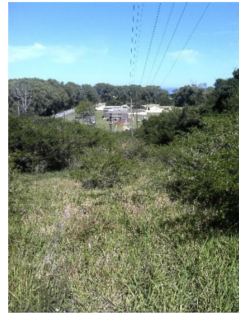
RM2: Seaview pump station complex and powerline servitude taken from the hill above the complex in the existing pipeline servitude. Also note powerlines Photo 34
