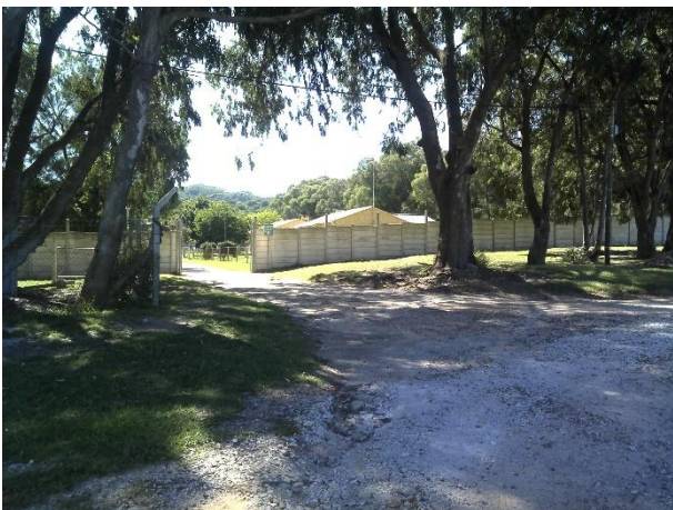
250 L Reservoir PS b: Entrance to the Seaview pump station complex – off the Seaview Road Photo 49
