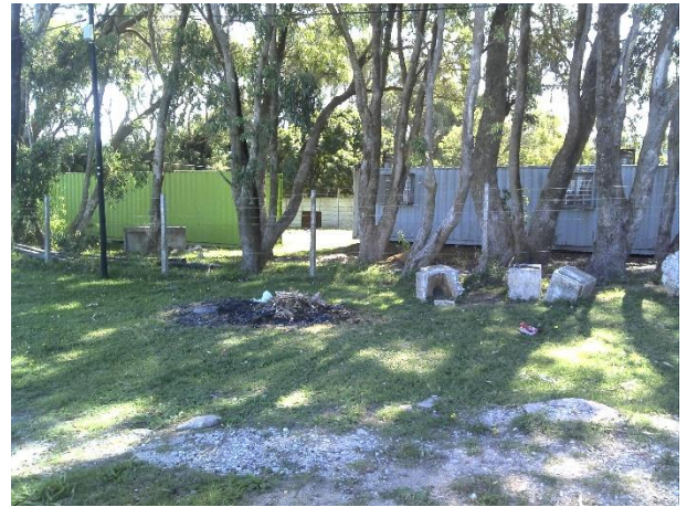
250 L Reservoir PS a: Boundary fence of the southern section of the Seaview pump station complex Photo 48
