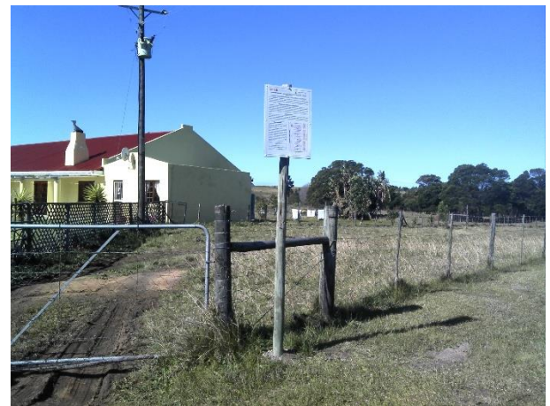
17g: Point where the pipeline alignment changes direction and runs along the existing municipal access road to the existing Greenbushes Reservoir. Note the project poster Photo 24
