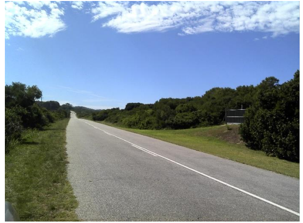
GM1-7: Option 1 pipeline alignment in the Seaview Rd servitude to the west of the road Photo 46
