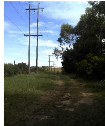
RM4: Access road along the existing pipeline servitude to the west of Seaview Rd Photo 32
