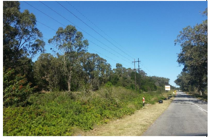
9g: Some areas within the road reserve are overgrown with vegetation that will need to be cleared. Note the powerline. Photo 14
